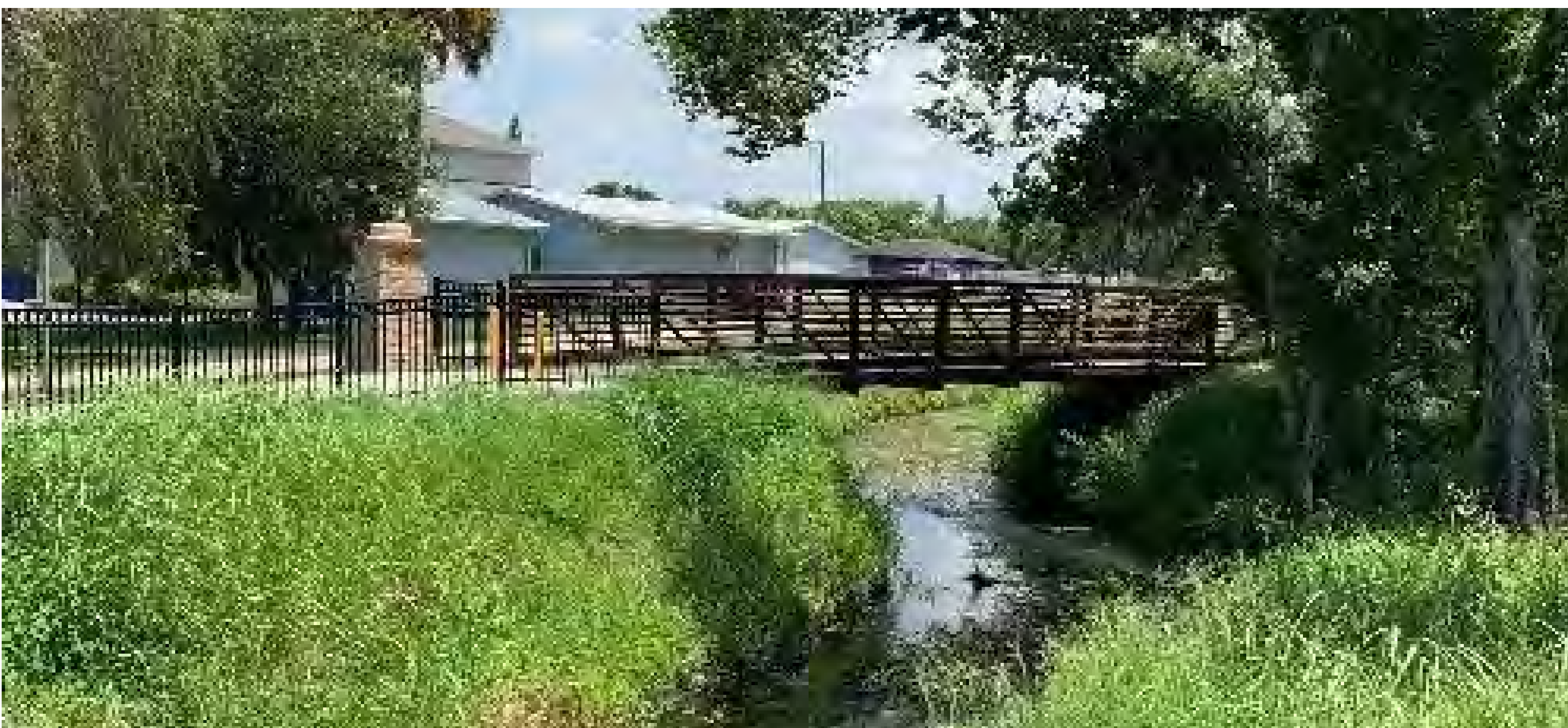
Prefabricated Steel Truss (Dr. Martin Luther King Jr. Trail)
