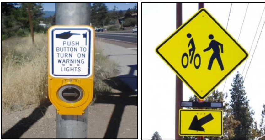
Figure 53. Push button activation of the rectangular rapid flashing beacon (left) and the beacon under the sign (right).
