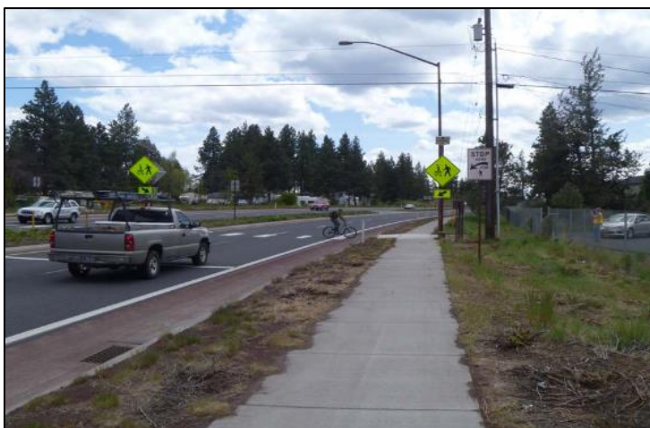
Figure 54. A rectangular rapid flashing beacon installation site in Bend, Oregon.
