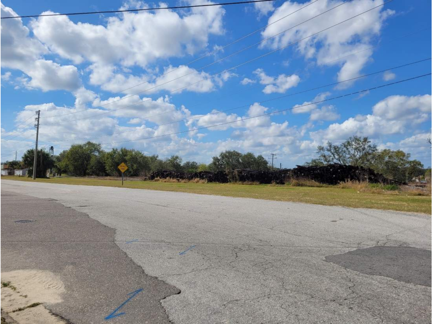
Segment 10: Looking west from the end of the proposed trail, pile of railroad ties observed in distance
