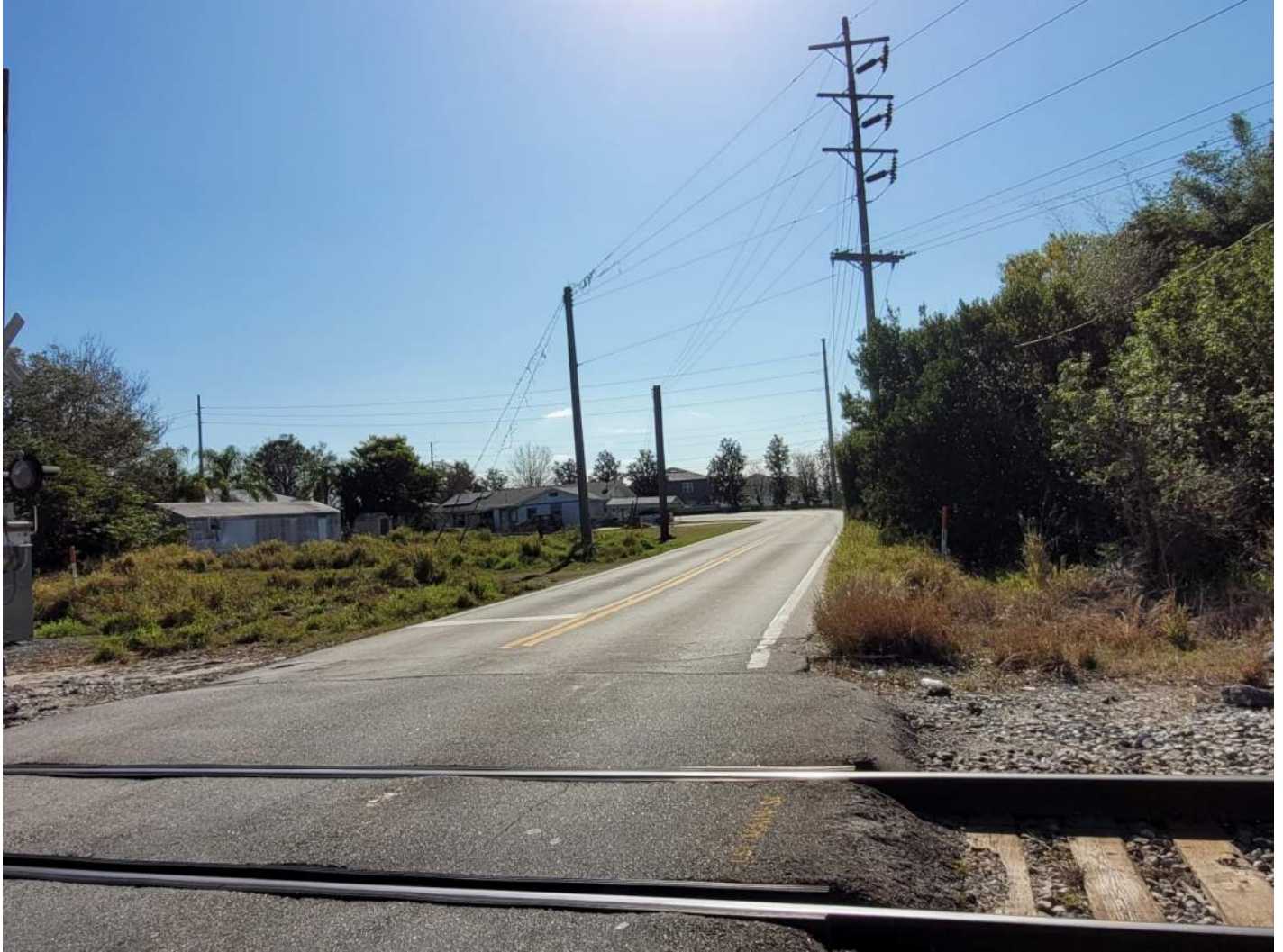
Segment 5: Looking southeast along West Pierce Street toward the railroad corridor intersection
