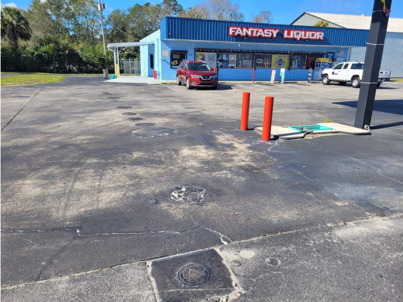
Map ID 4: Multiple monitoring wells located throughout the site
