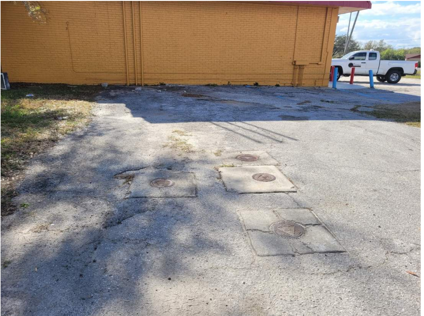
Map ID 17: Multiple monitoring wells located throughout the site
