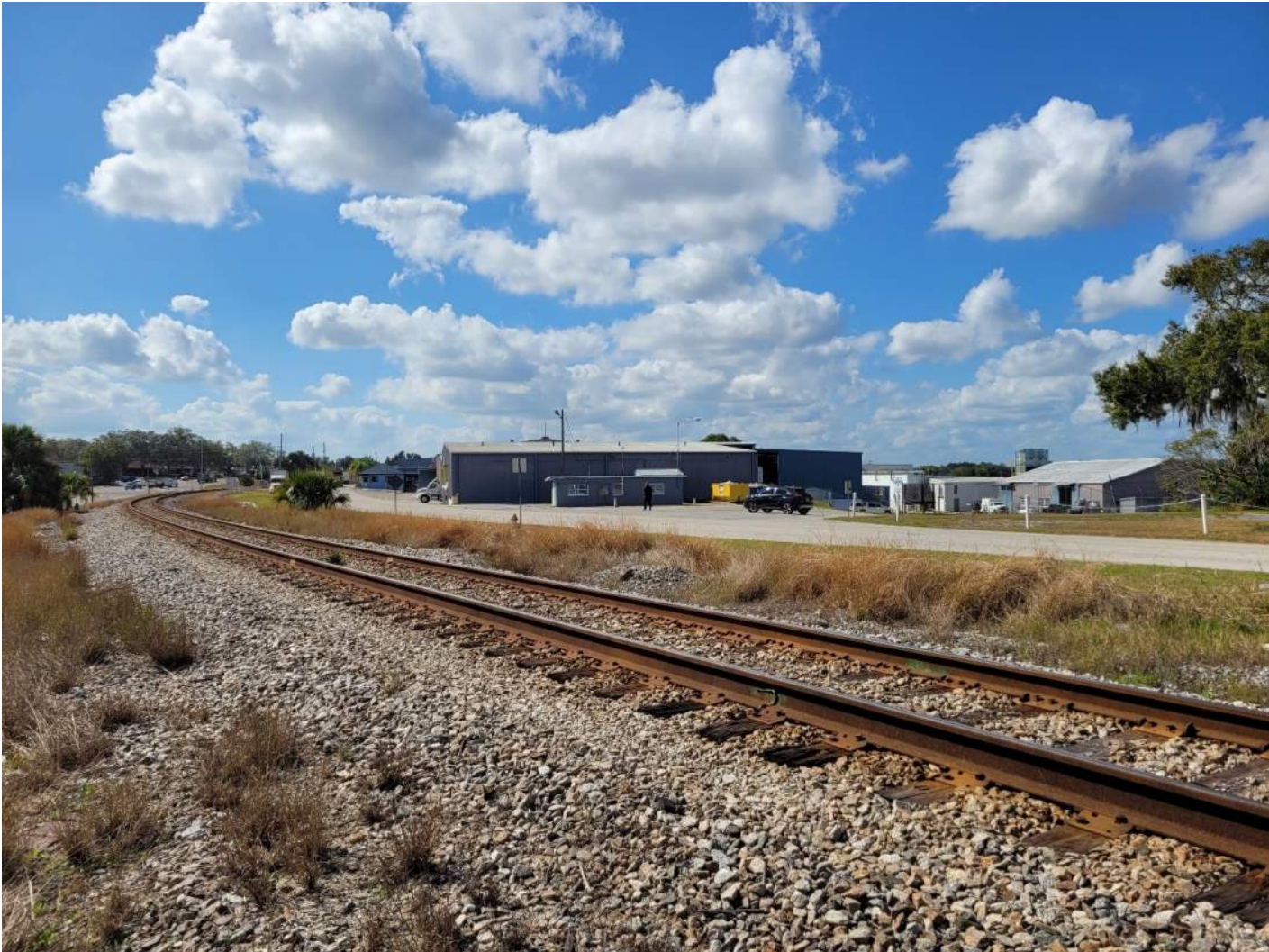
Segment 10: Looking southwest along the railroad corridor
