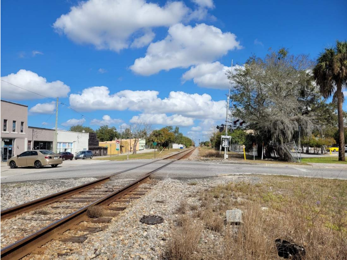
Segment 10: Looking northeast along the railroad corridor
