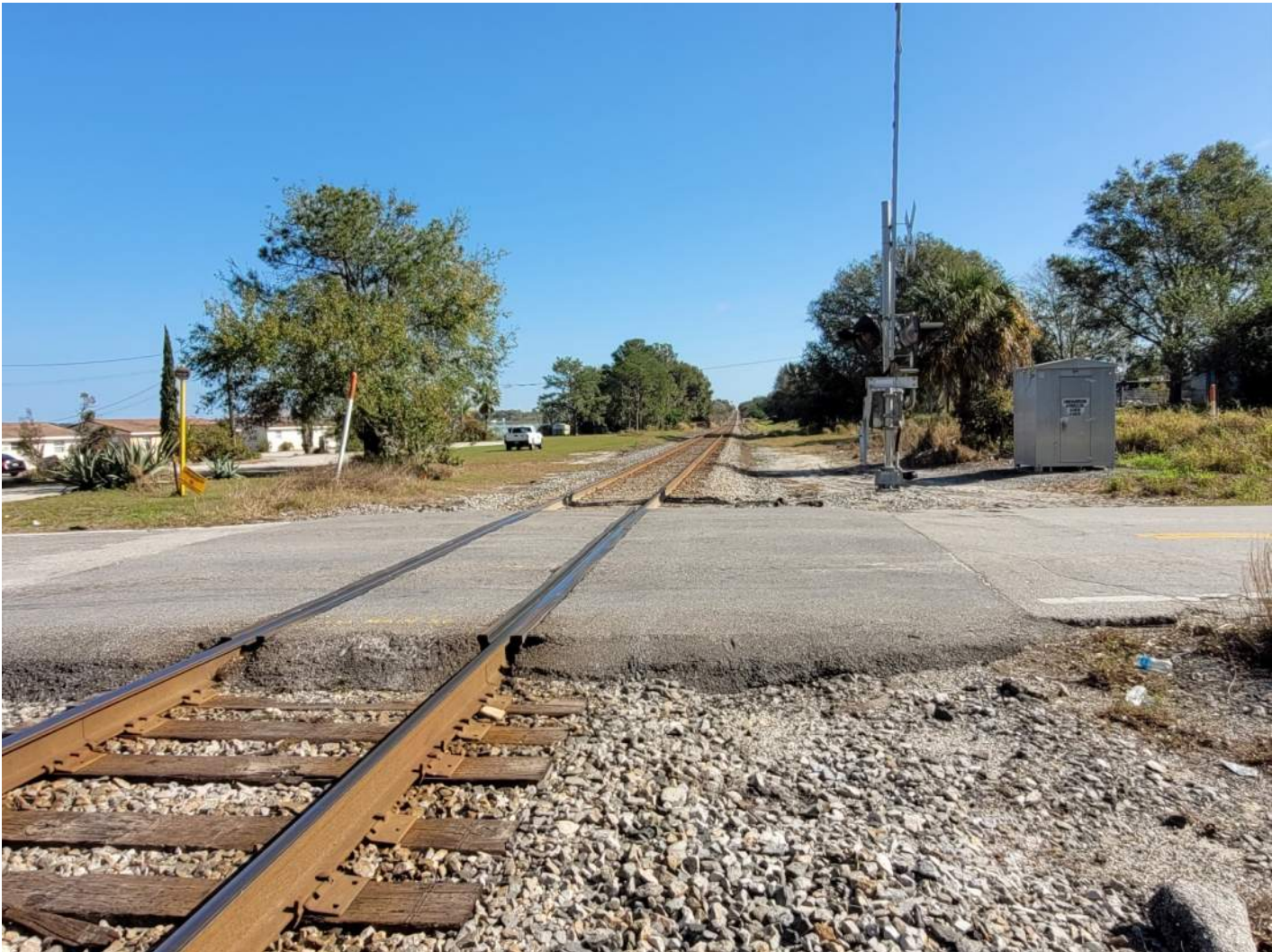
Segment 5: Looking northeast along the railroad corridor
