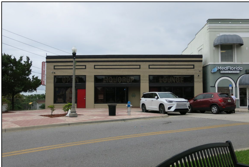
Photo 2 - 600-604 Ingraham Avenue E (8PO02881), looking north.
