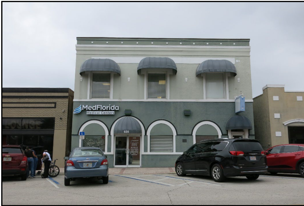
Photo 1 - 606-608 Ingraham Avenue E (8PO02880), looking north.
