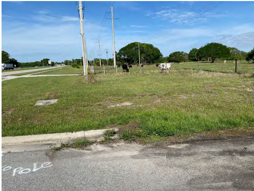
Survey Station No. 5 – Facing West
