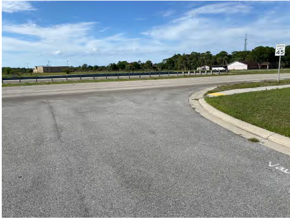
Survey Station No. 5 – Facing South
