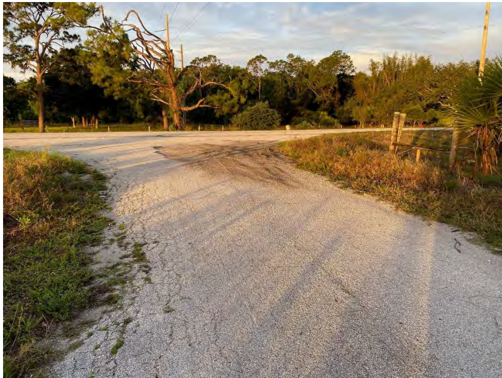
Survey Station No. 6 – Facing West
