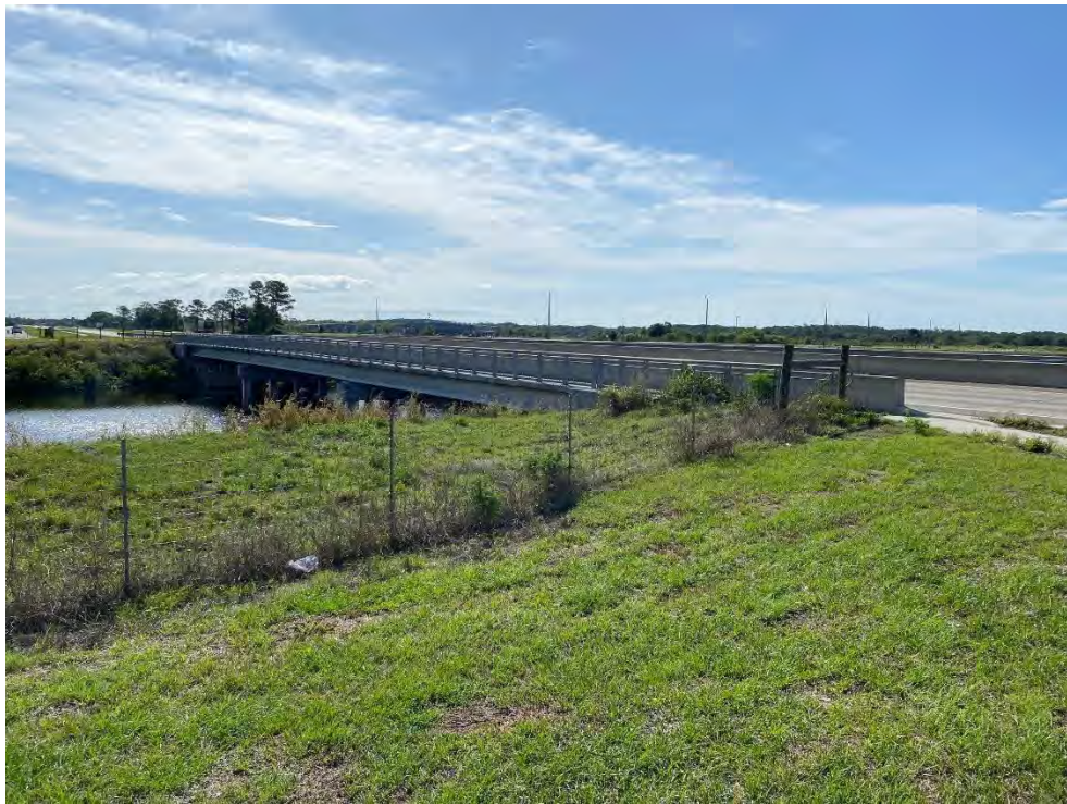
Survey Station No. 5 – Facing East
