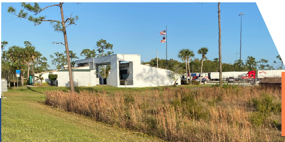
Lee County Rest Area Building
