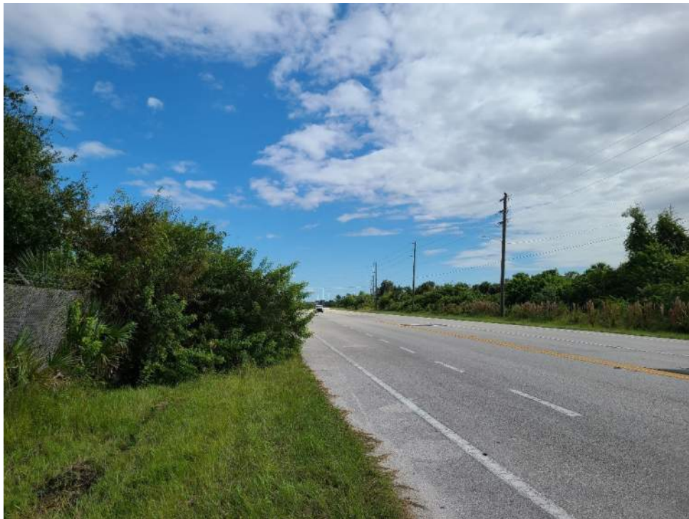
Near the eastern project boundary Harborview Road looking northwest
