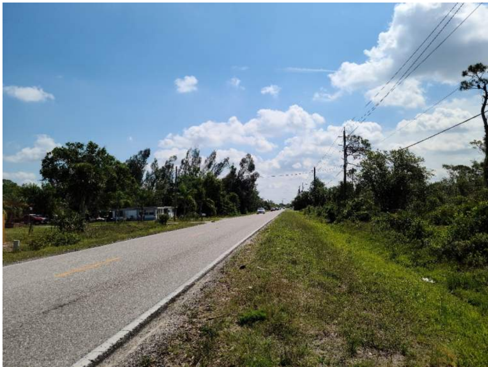
Sapodilla Street and Harborview Road Near the eastern project boundary looking east
