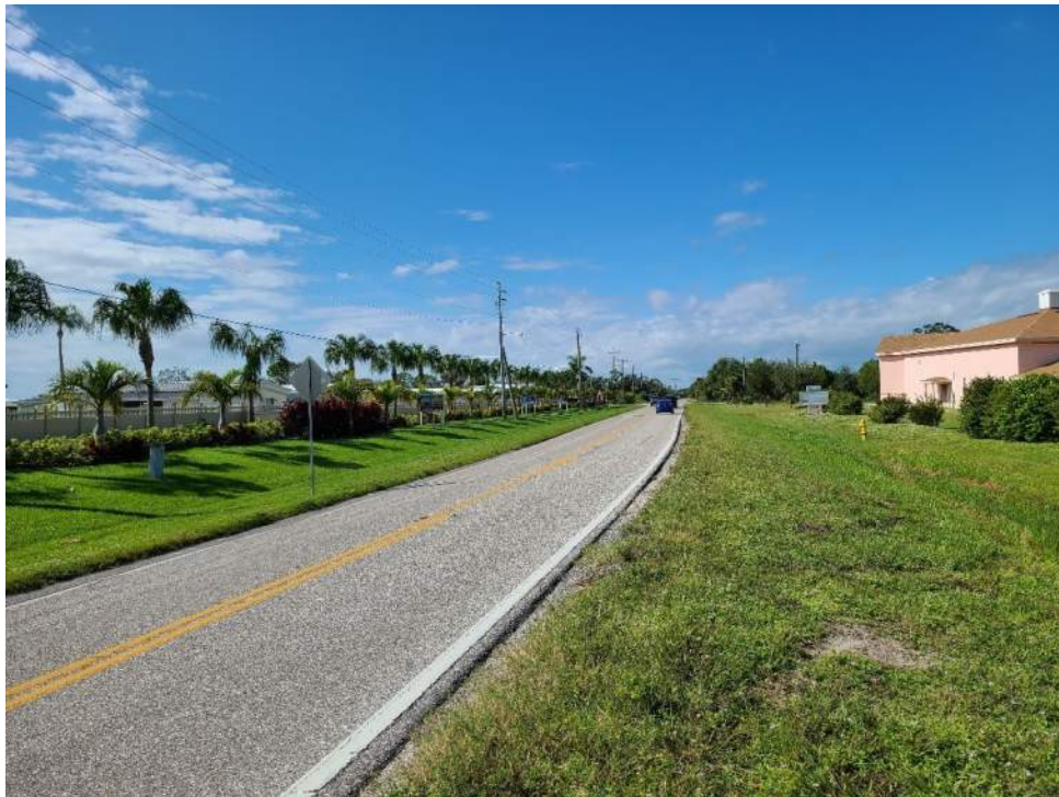
Near the center of the project Harborview Road looking southwest
