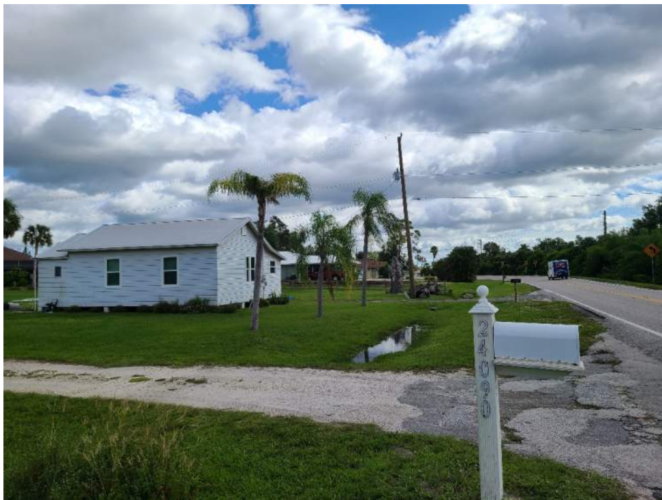
SMF 1-2B Looking east
