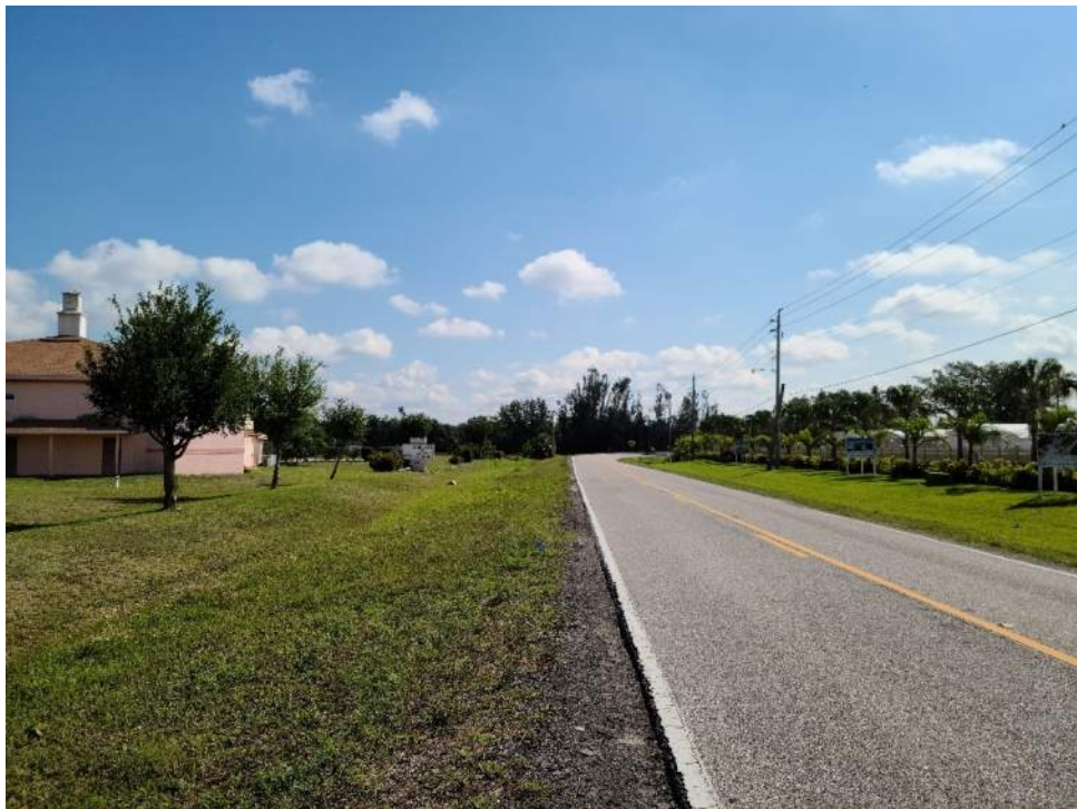
Rowland Drive and Harborview Road Near central portion of the project looking northeast
