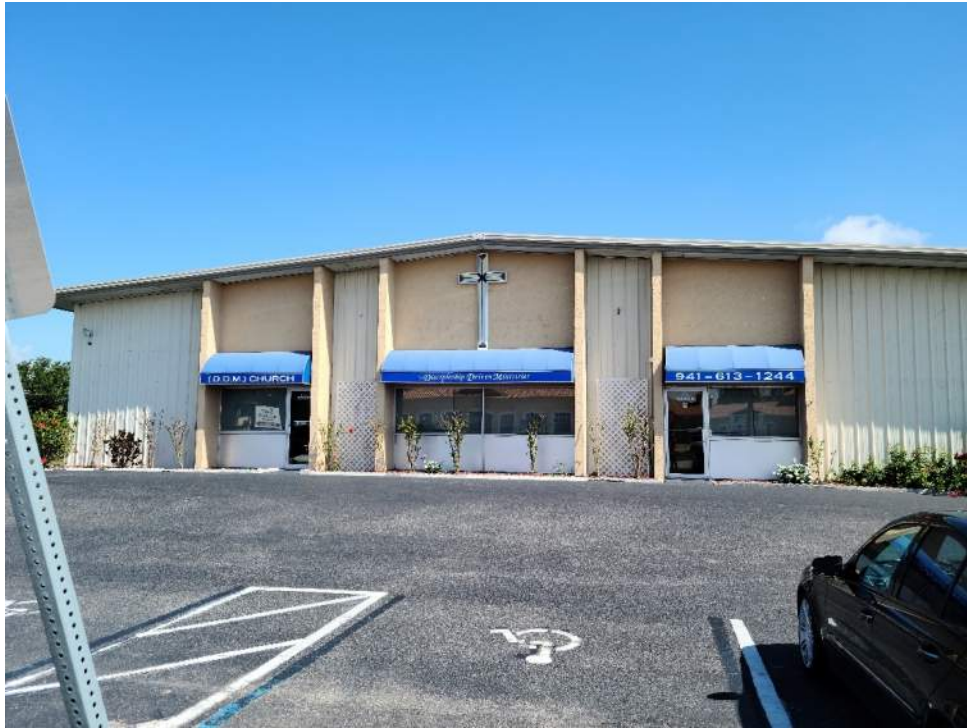
Site 1 – Former Marketing Arm International Harborview Road looking north
