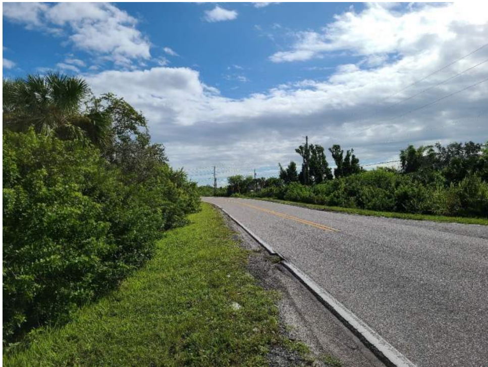
Near the eastern project boundary Harborview Road looking east
