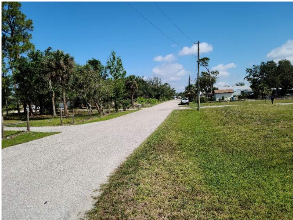
Cortez Drive Near western project boundary looking north
