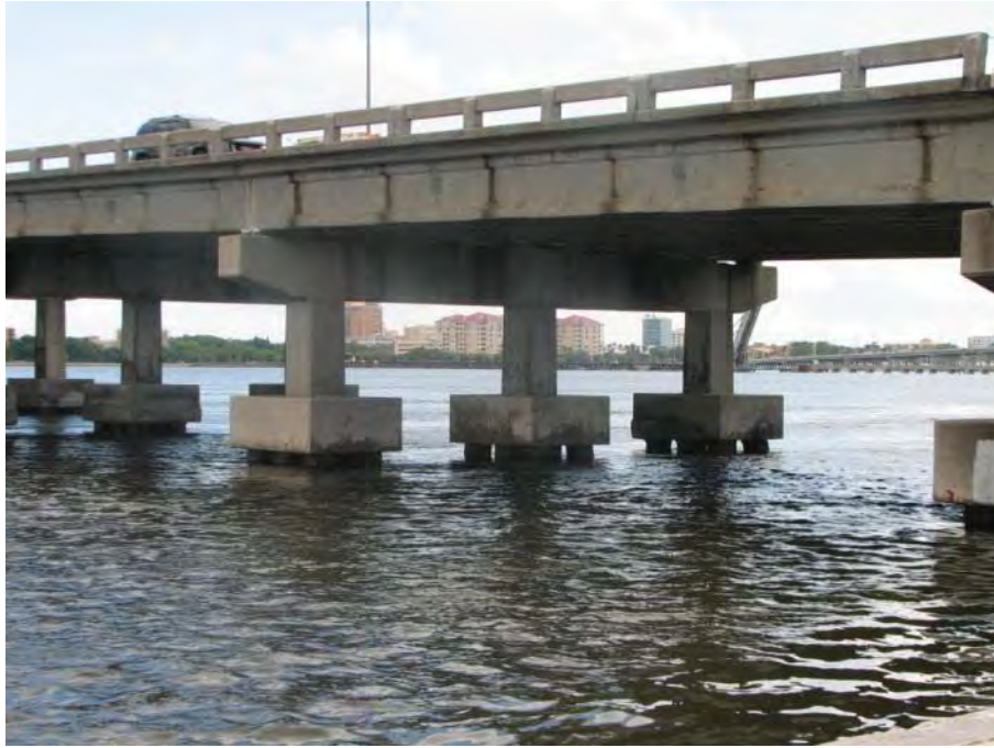
Homogeneous Material E – Various concrete elements
