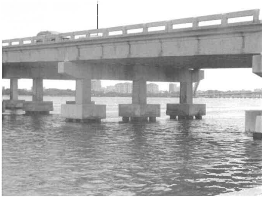
Homogeneous Material E – Various concrete elements
