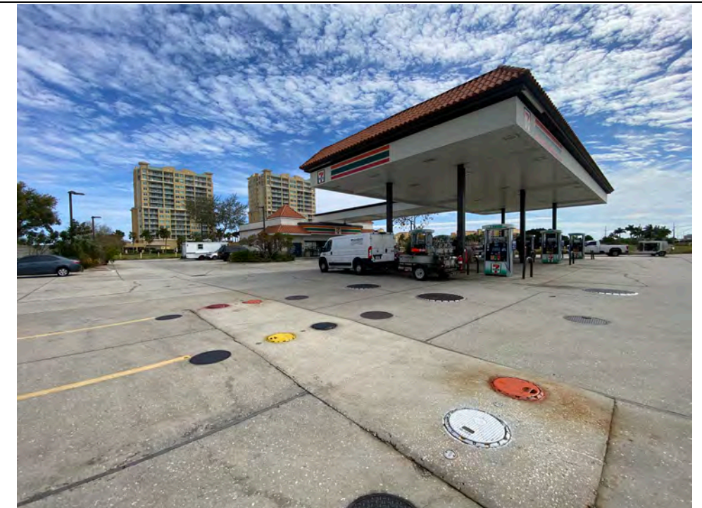
View of the existing gas station from the northwest corner of the facility, facing southeast.
