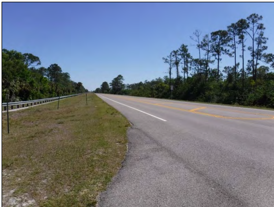
FIGURE 9-51 STATE ROAD 29 (8CR1309), C. 1925, CONSIDERED NATIONAL REGISTER-INELIGIBLE, FACING SOUTHEAST
