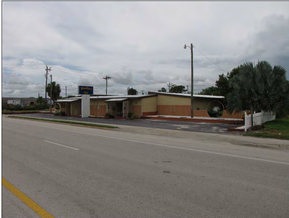
FIGURE 9-71 BUDGET INN/504 MAIN STREET E (8CR1370), C. 1950, CONSIDERED NATIONAL REGISTER-INELIGIBLE, FACING NORTHWEST
