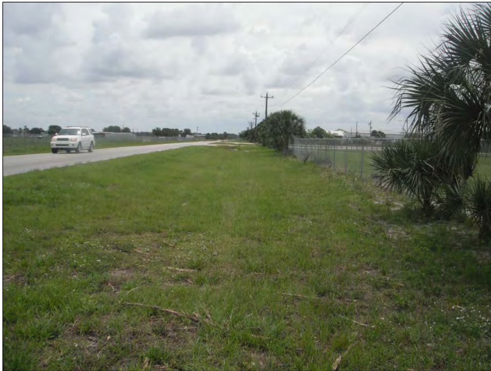
FIGURE 9-1 SOUTHERN CR 846 ROW WITH DITCH AND BERM, BURIED AND OVERHEAD UTILITIES, FACING EAST
