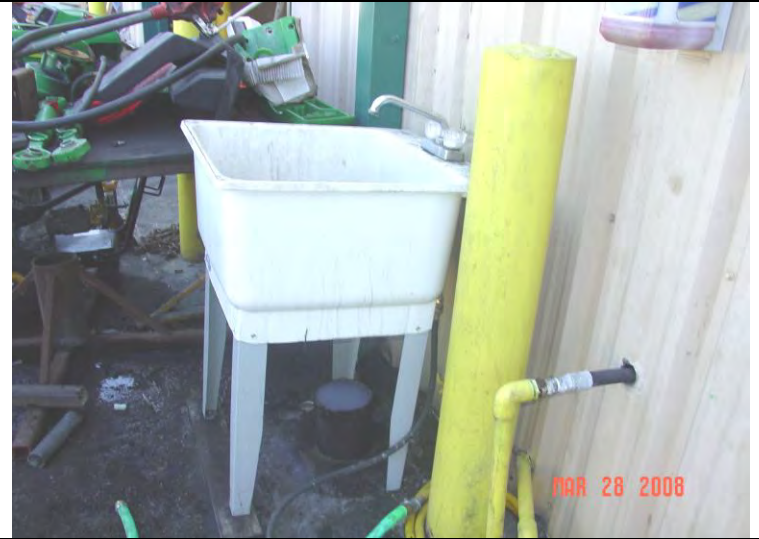
Photo 1 - Hand washing sink not connected to sewer
