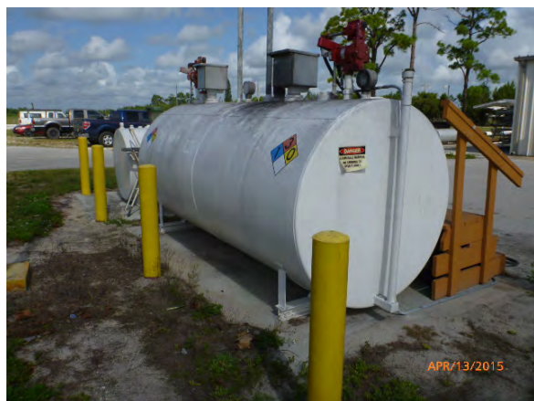
2015-04-13 TCI Inspected AST system
