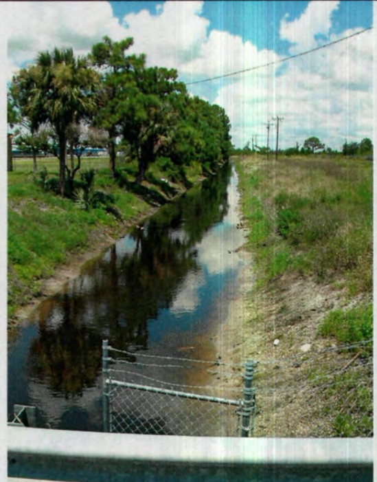
Ditch looking north toward packinghouse and well.
