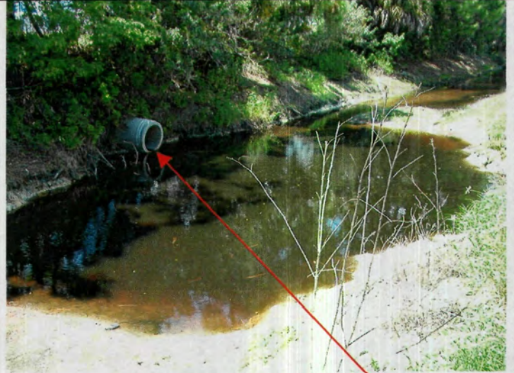
Market main storm water outfall.
