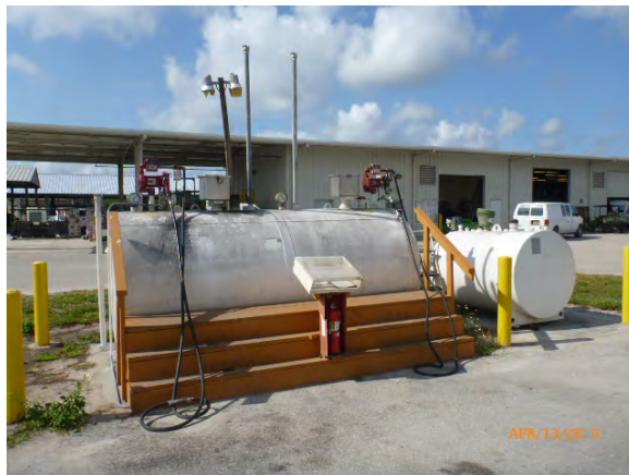
2015-04-13 TCI Regulated (L) and unregulated (R) ASTs
