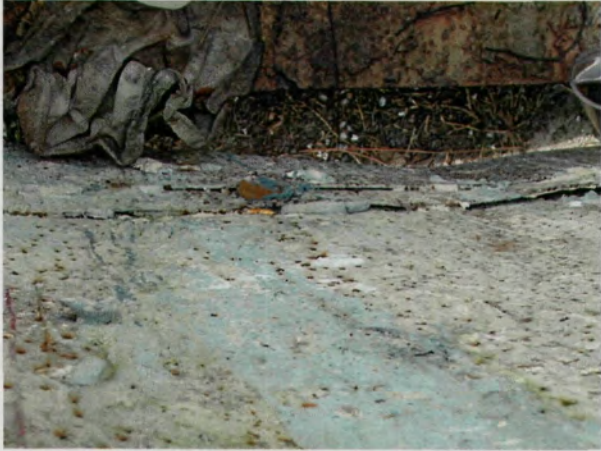
Bottom of dumpster split wide open.
