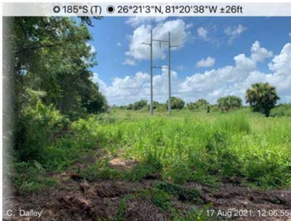
Photo 3: Electric Utility Corridor
