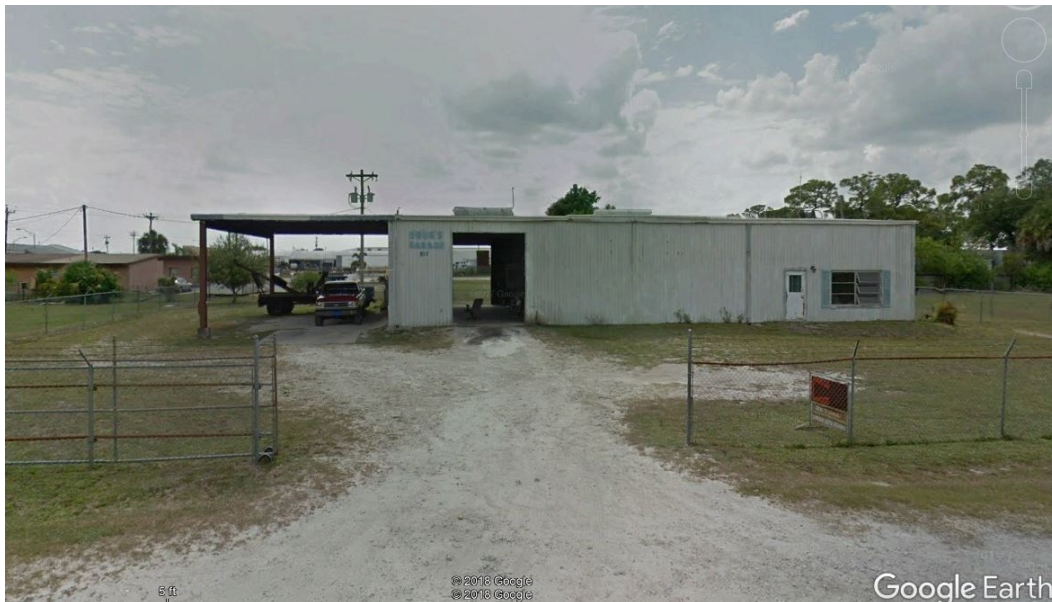
517 New Market Road — Repair Shop
