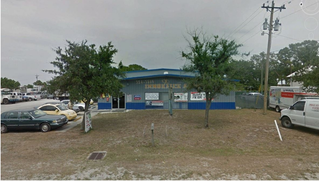
524 New Market Road — Rental Facility
