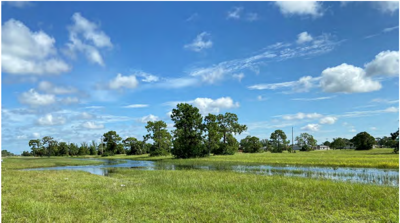
Photo 5. Ditch leading to a cross drain on the east side of the roadway, photo taken during the wet season in September 2020. Water overtops the embankment and floods the roadside edge.
