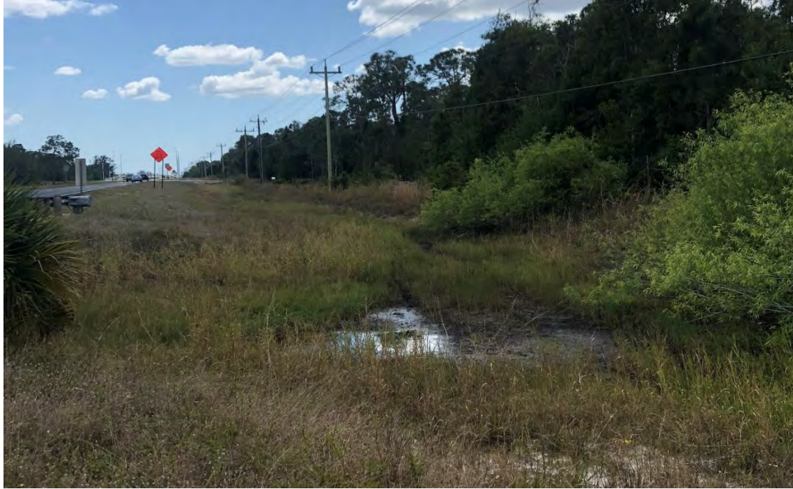
Photo 3. Ditch leading to a cross drain on the west side of the roadway, photo taken during the dry season in March 2020.
