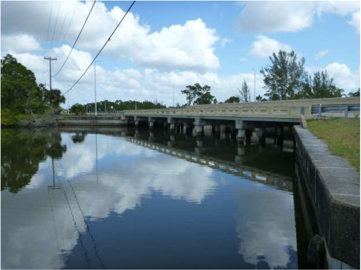
Bridge piers looking from southwest bank facing north
