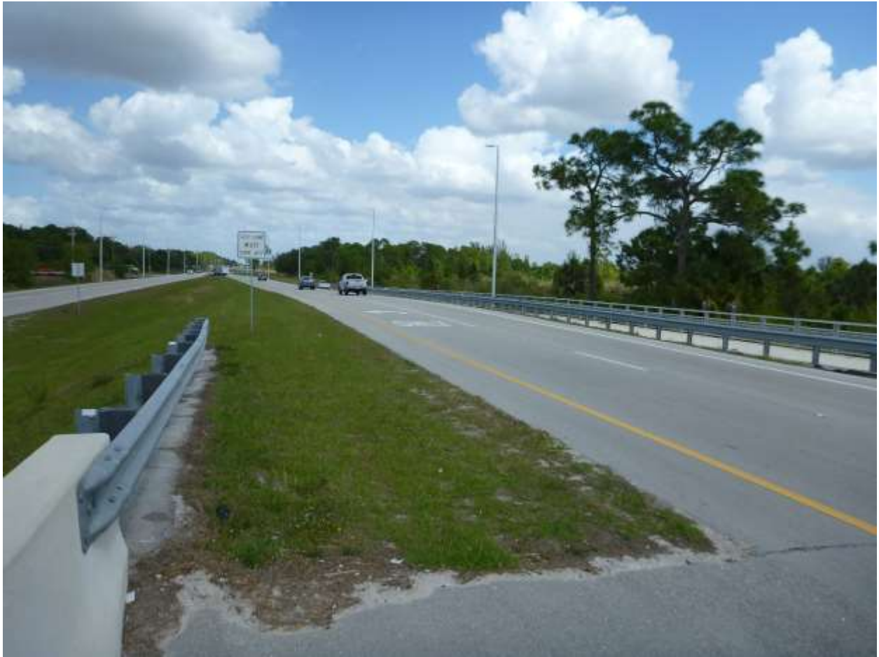
North approach from northwest side
