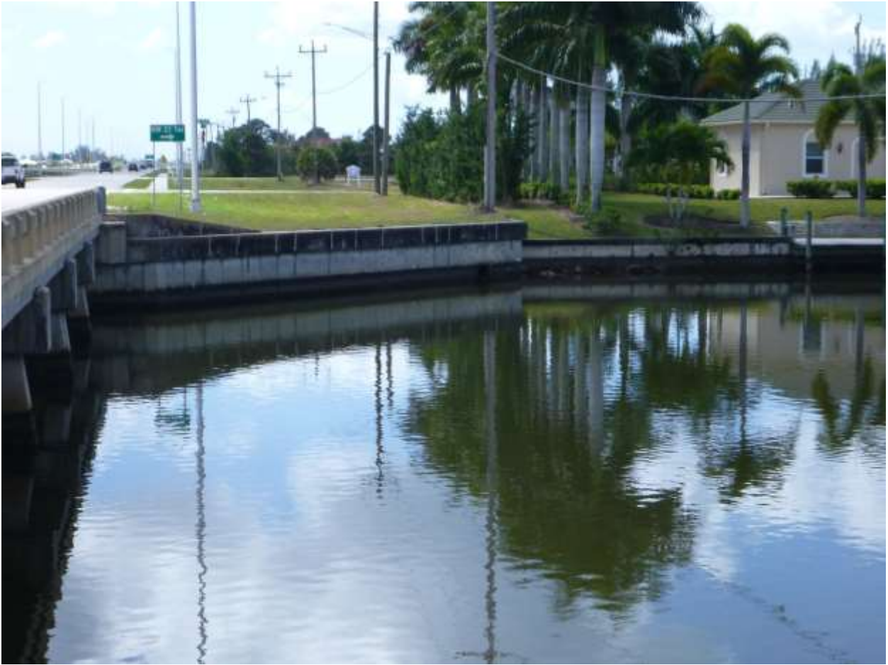
Southwest bank and seawall
