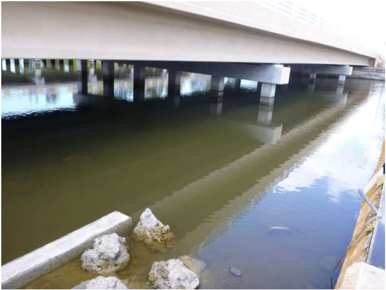
Piers looking from southeast to the north
