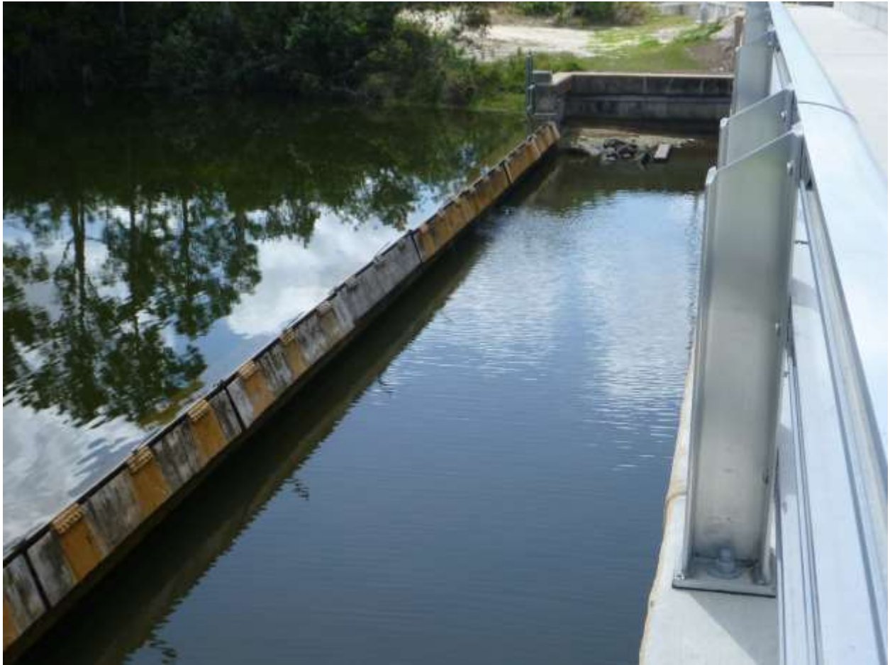
Weir looking south
