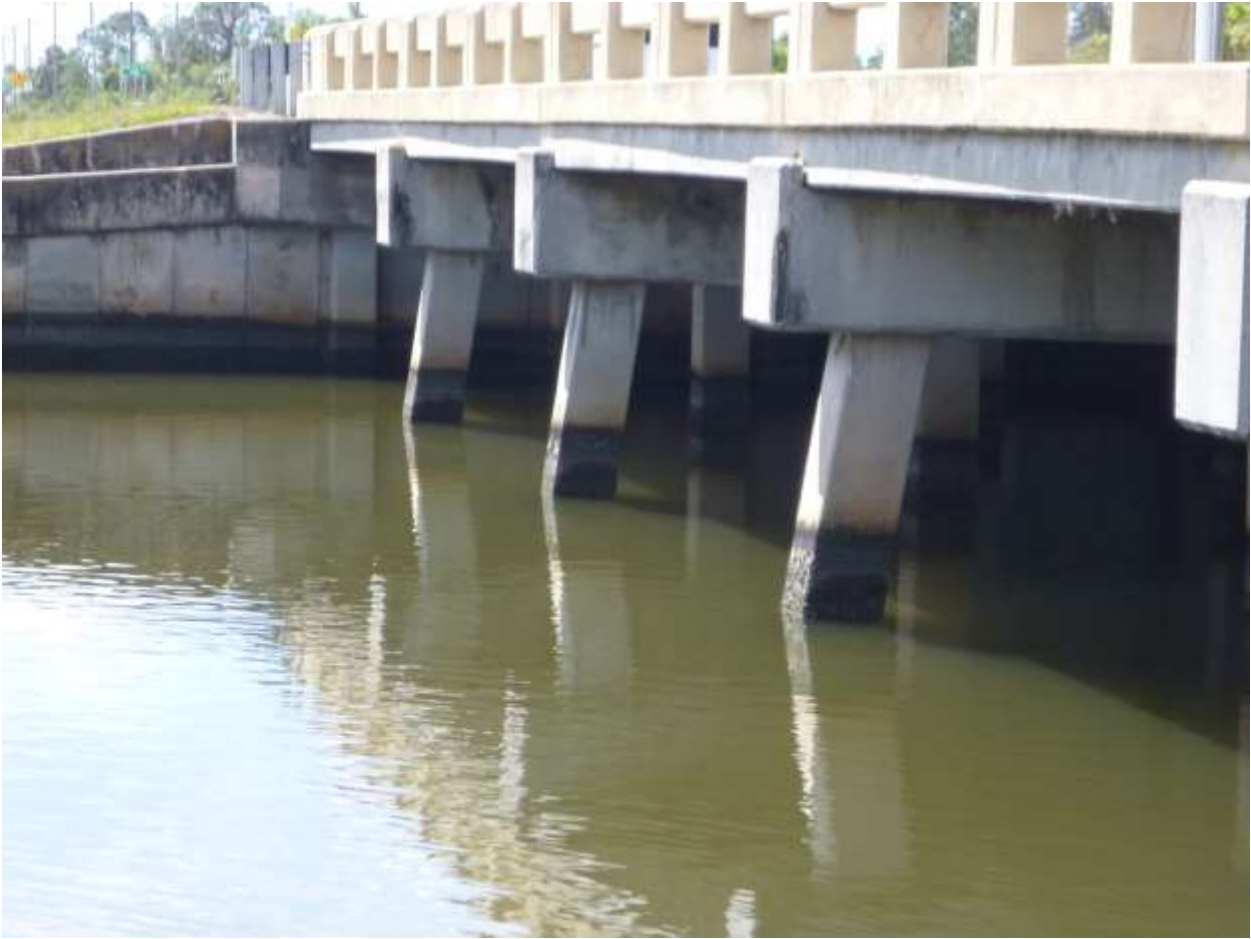
Southeast abutment and wingwall looking from northeast bank
