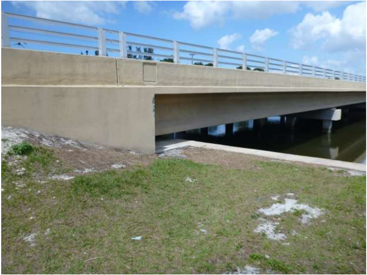
Southeast bank and abutment
