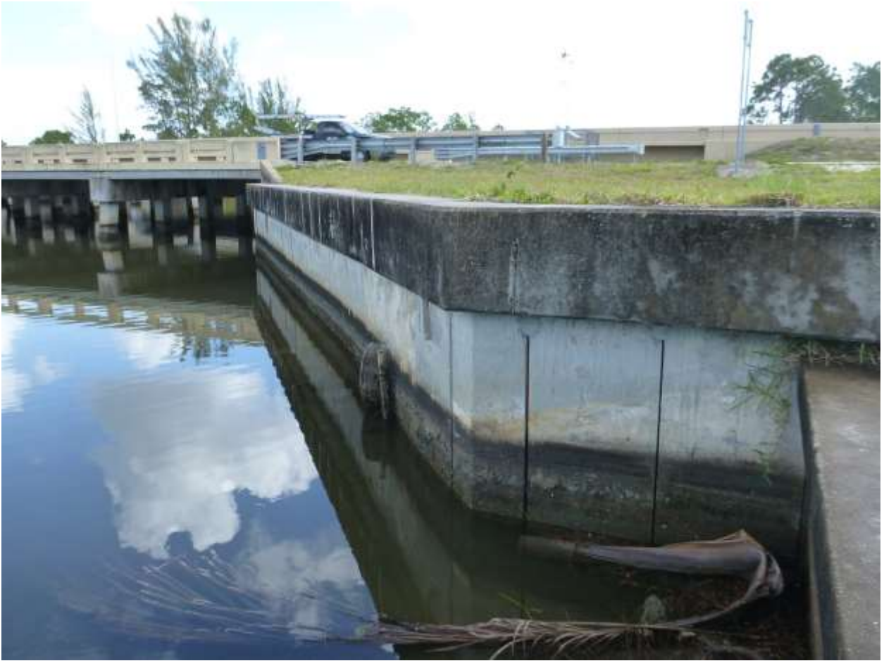
Southwest abutment and seawall
