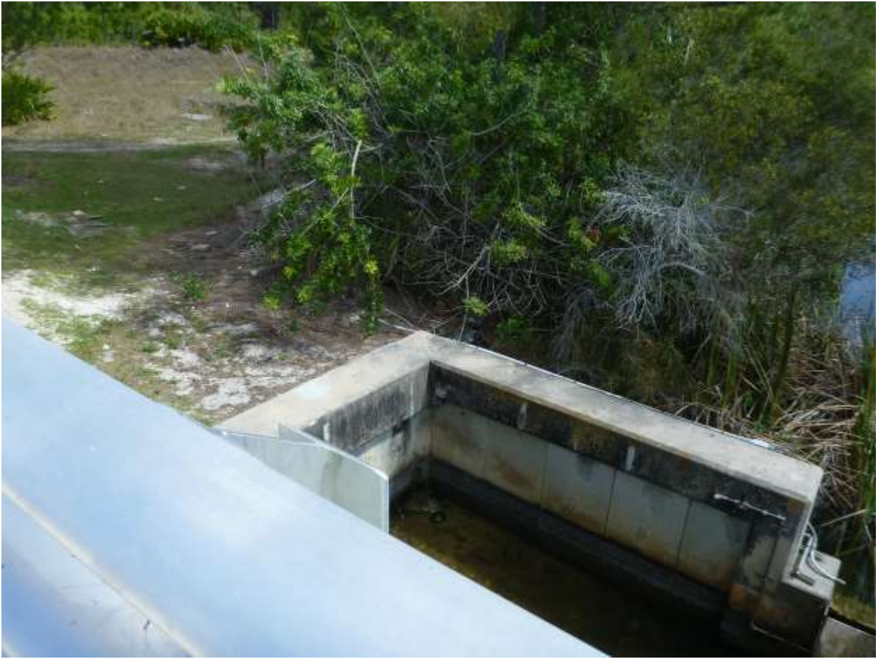
Northeast bank and wall
