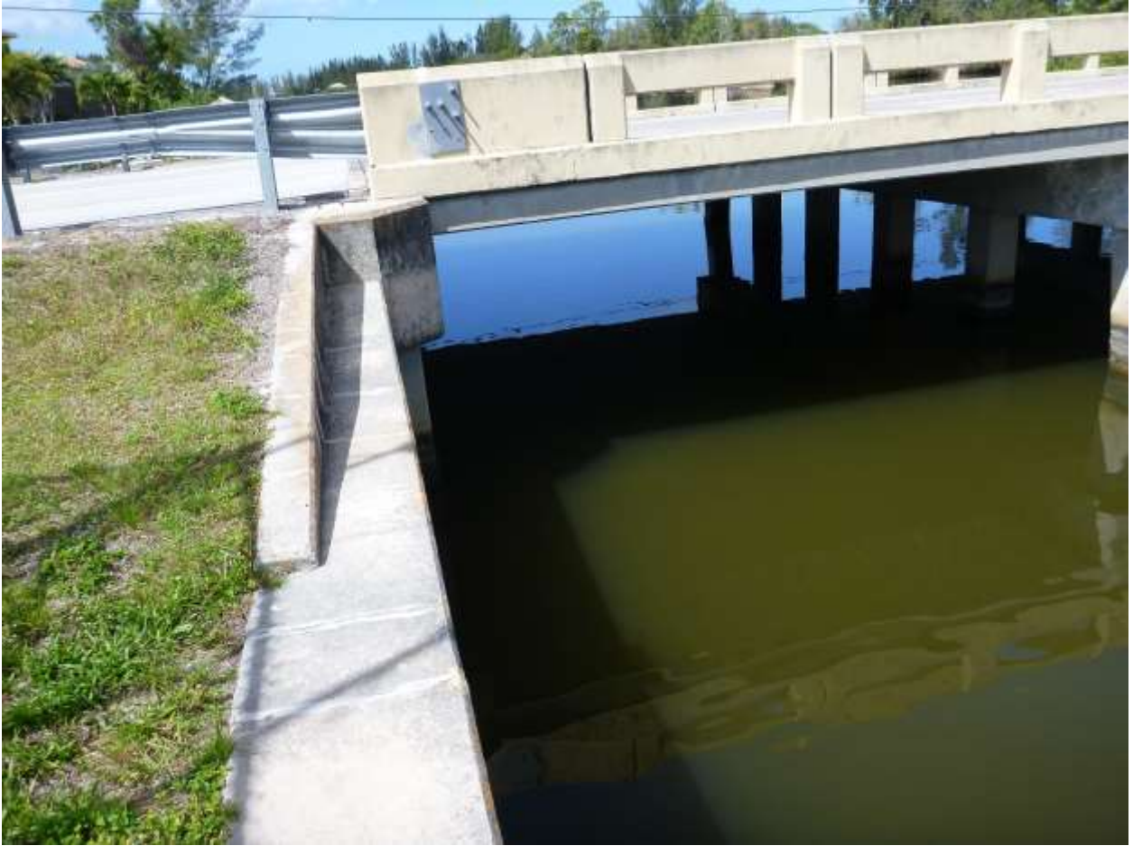
Southeast abutment and seawall
