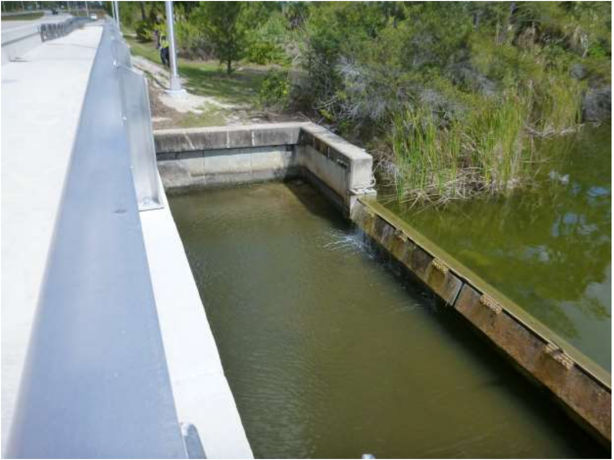
Weir, northeast bank
