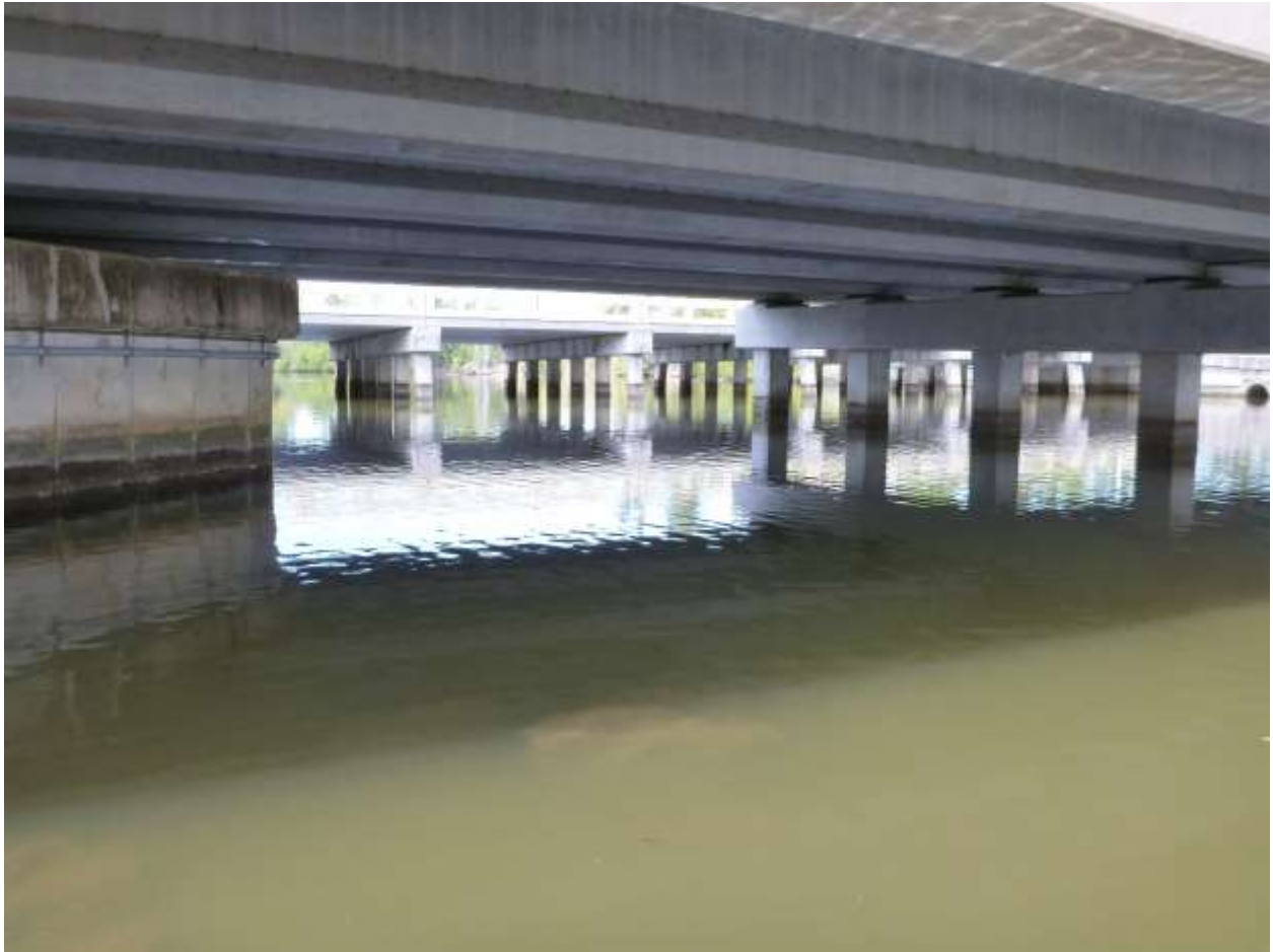
Abutment and piers
