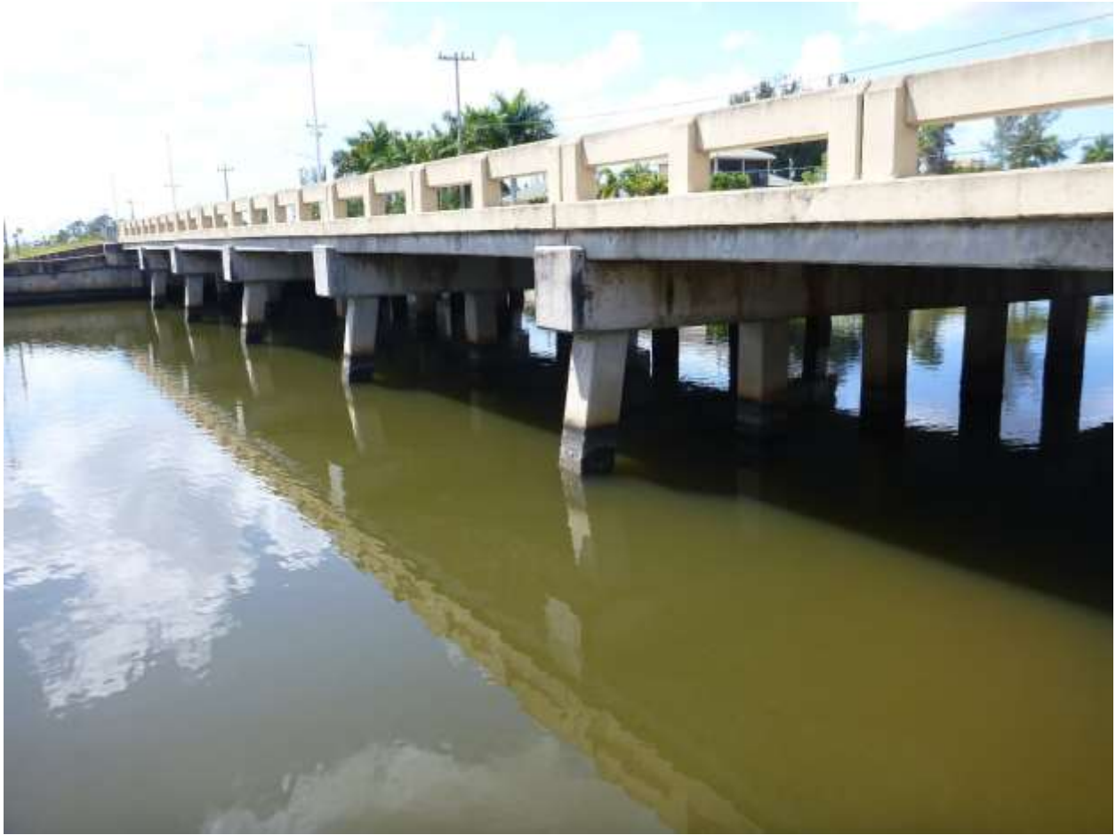
Bridge piers looking south
