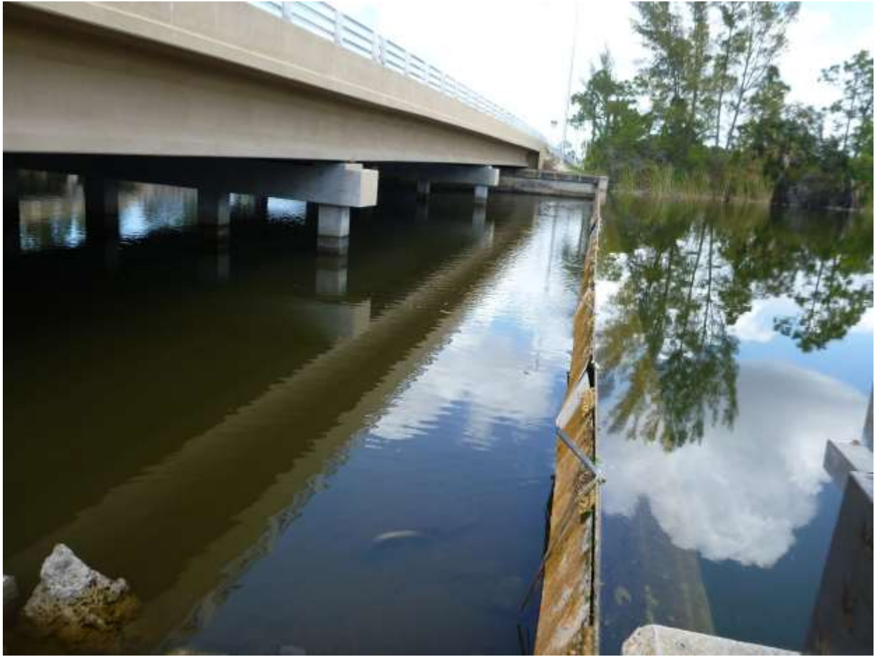
Weir looking north
