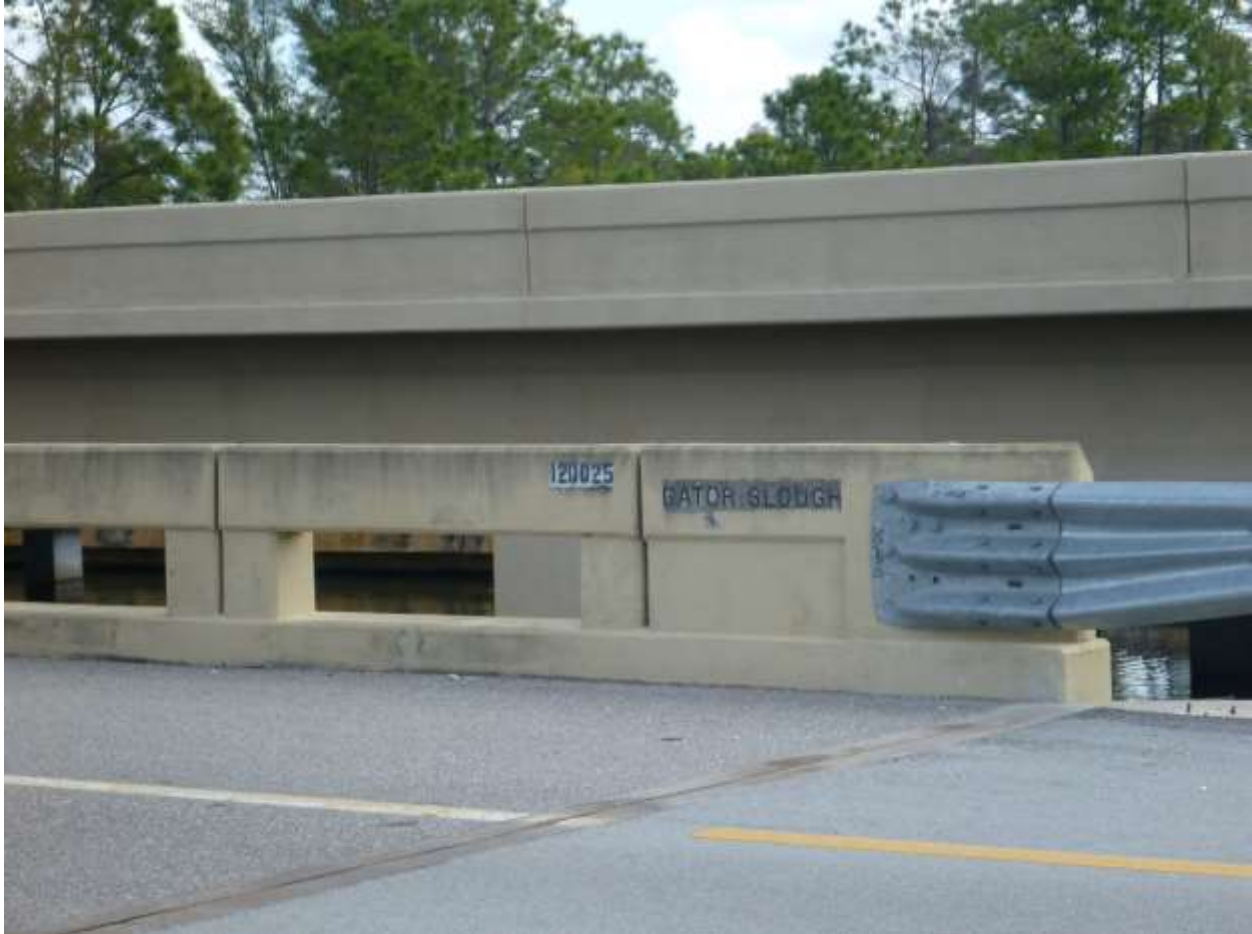
Bridge 120025 bridge number
