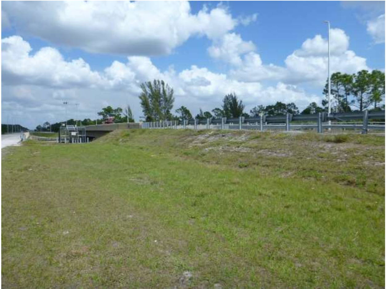
Area between two bridges facing north
