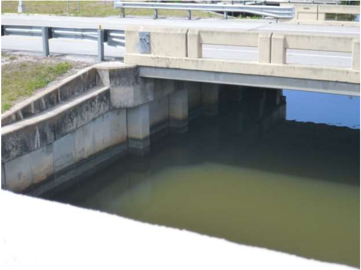
South abutment and seawall
