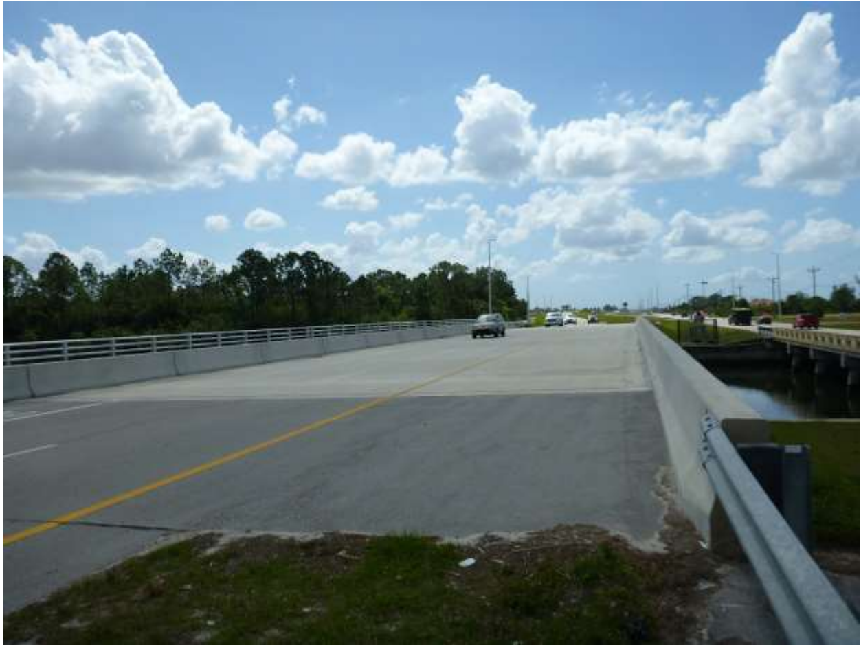
Bridge roadway looking south from northeast side
