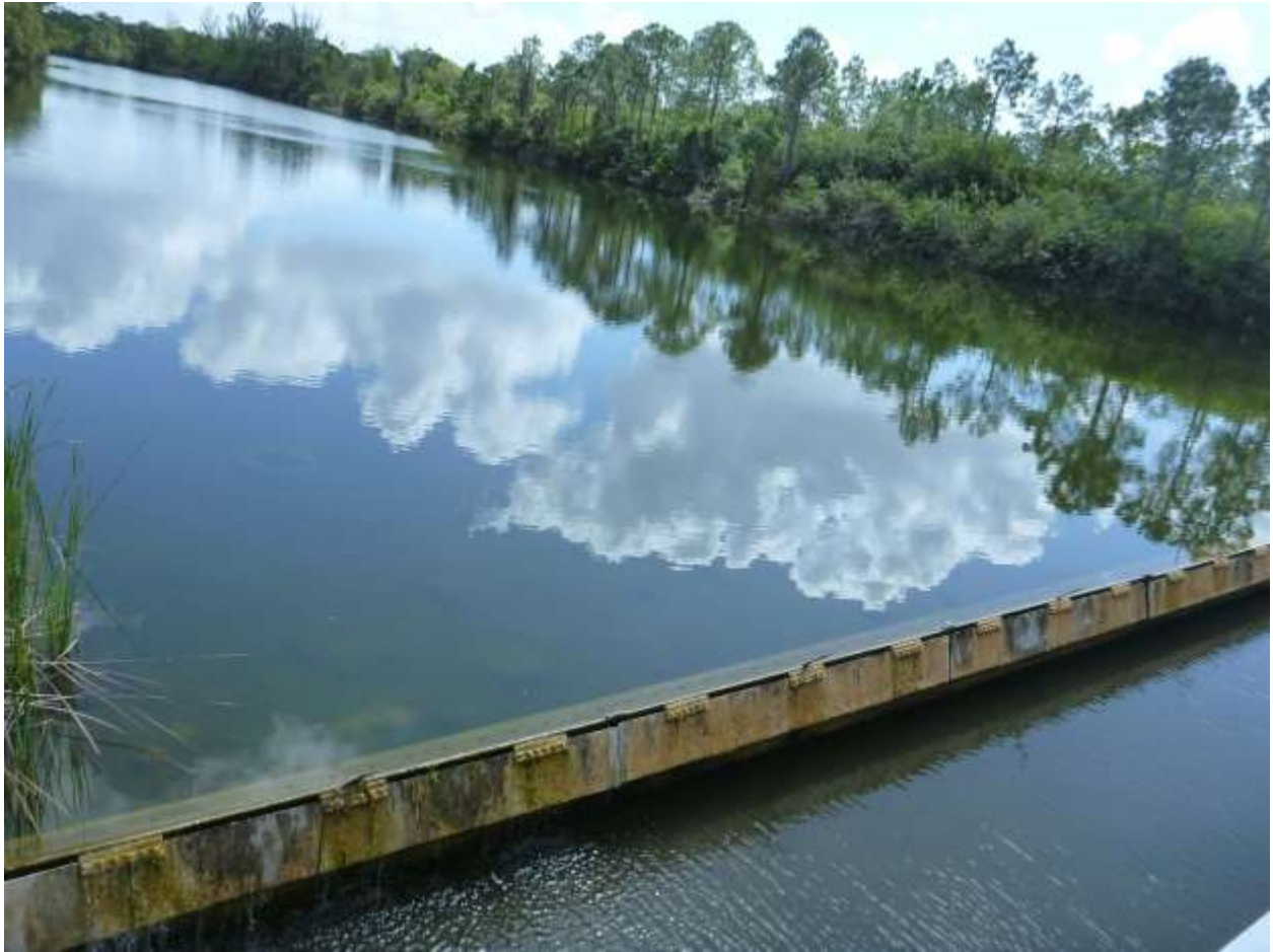
Weir looking southeast
