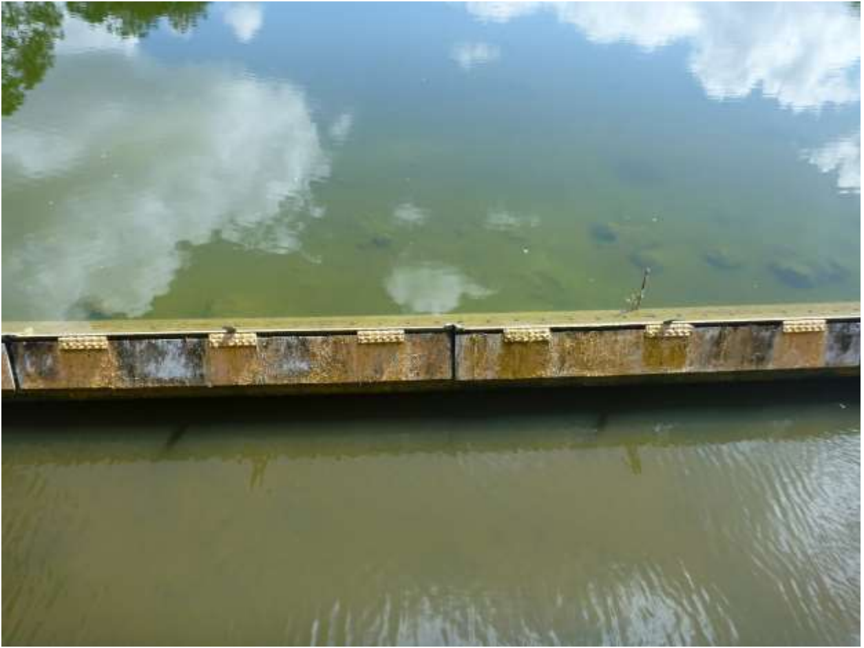
Weir looking east
