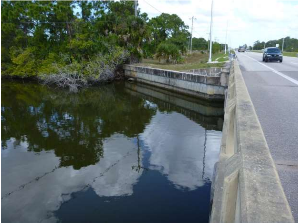
Northwest bank and abutment
