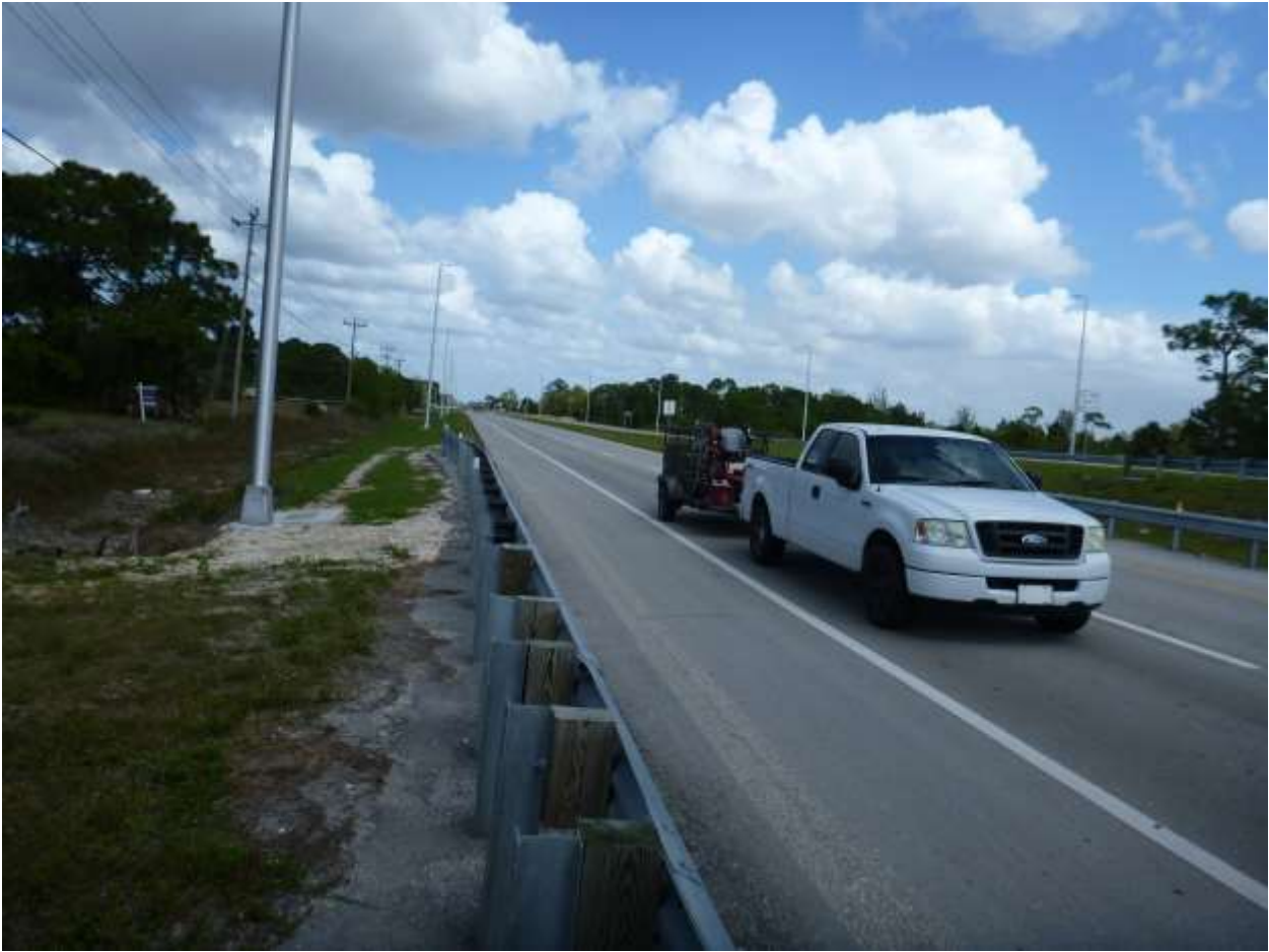
North approach looking from northwest bank
