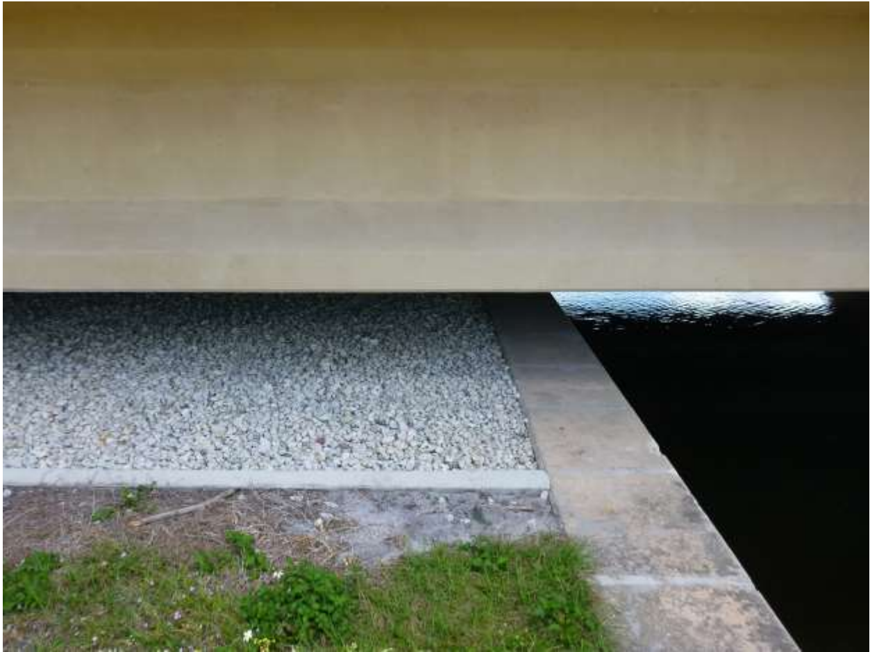
Northwest abutment and bank
