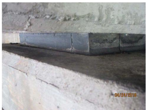
Homogeneous Area 1 (Samples 001-003) - Black bearing pad; between girder and end bent
