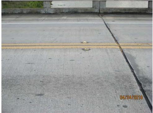
Homogeneous Area 6 (Samples 016-018) – Black reflector mastic; deck
