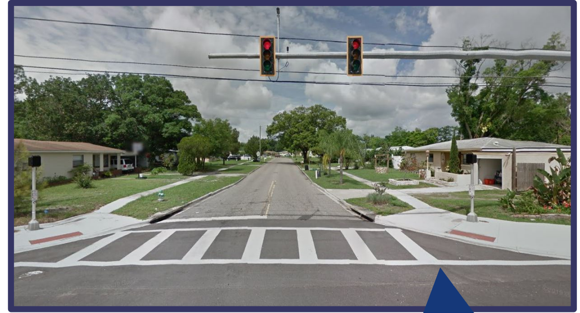
“Ladder” pattern crosswalk
