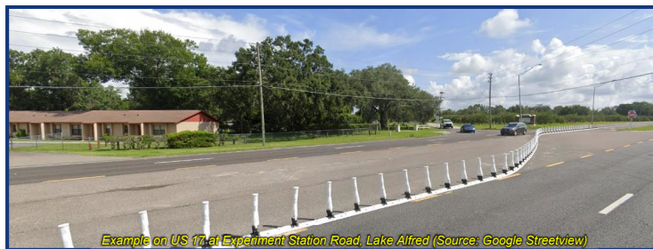
Example of a Directional Median Opening
