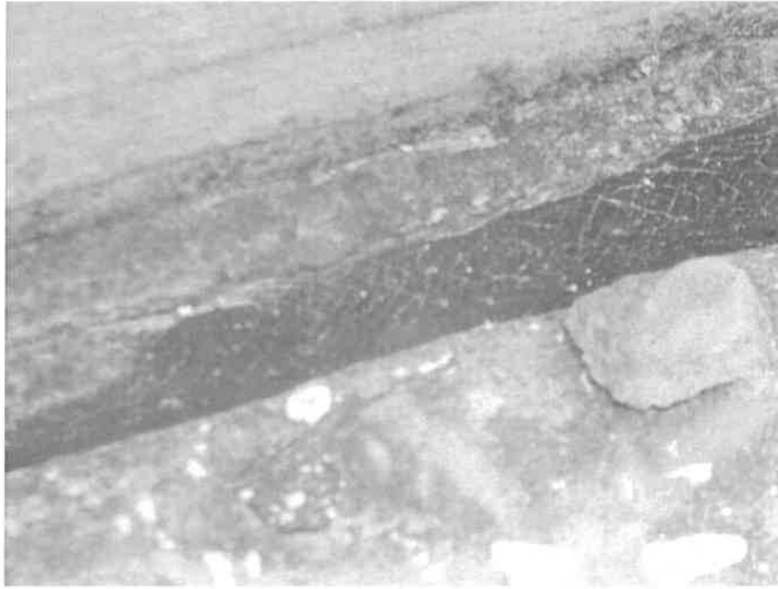
Homogeneous Material C – Poured joint filler at expansion joints on decking
