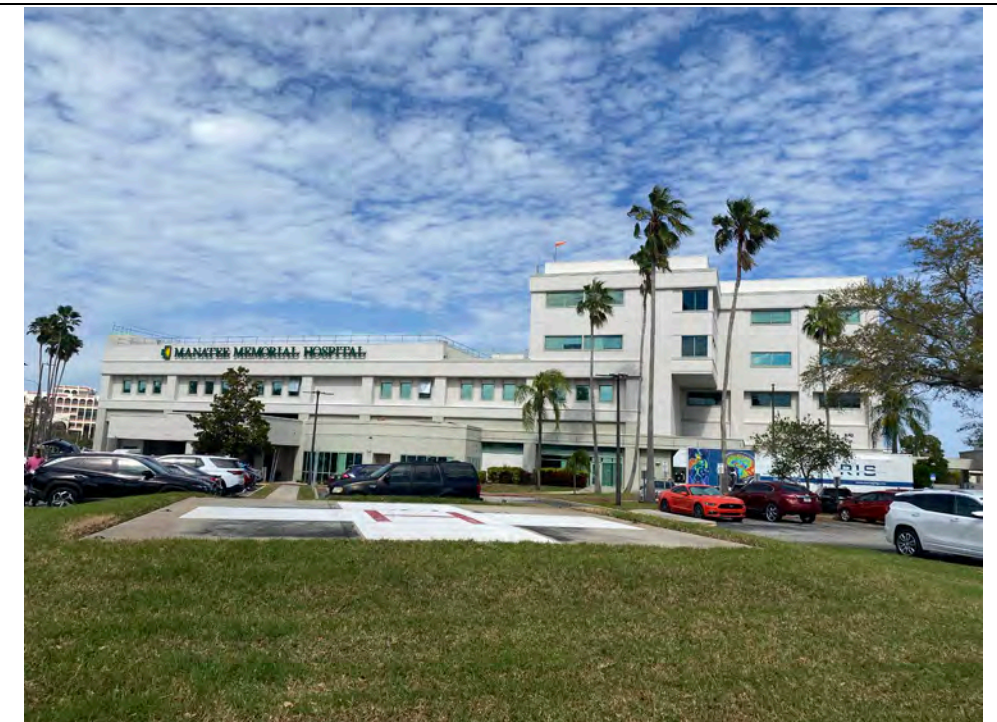
View of the southern portion of the Manatee Memorial Hospital building, facing north.
