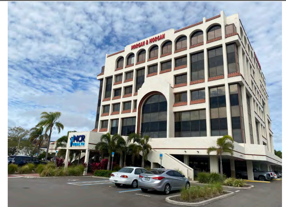
View of the multi-tenant professional office building, facing north.
