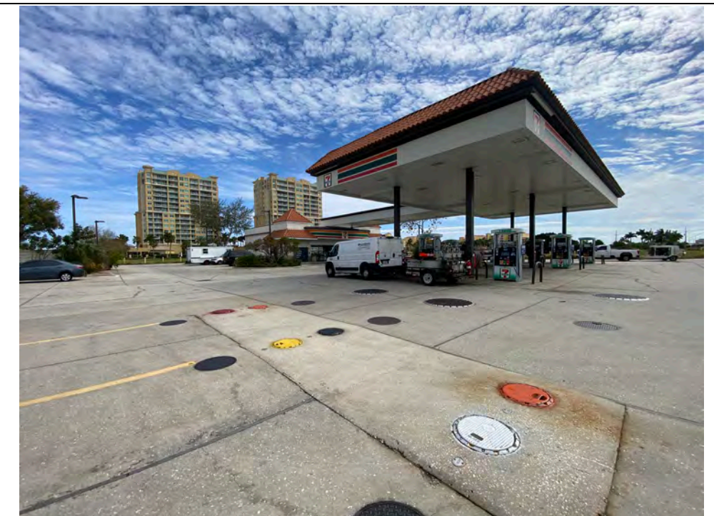
View of the existing gas station from the northwest corner of the facility, facing southeast.
