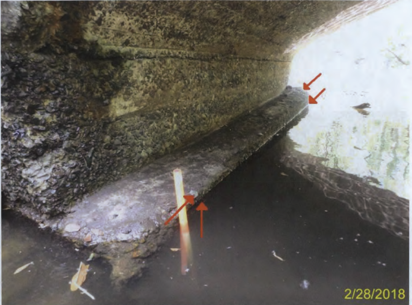
Photo 5 - Element 220 Re Conc Pile Cap/Ftg
