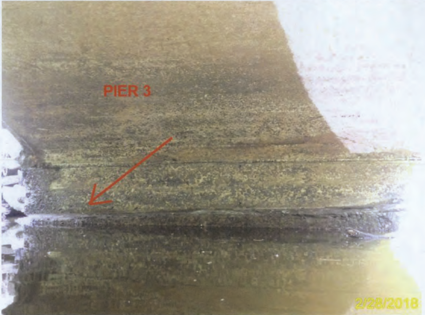
Photo 6 - Element 220 Re Conc Pile Cap/Ftg
