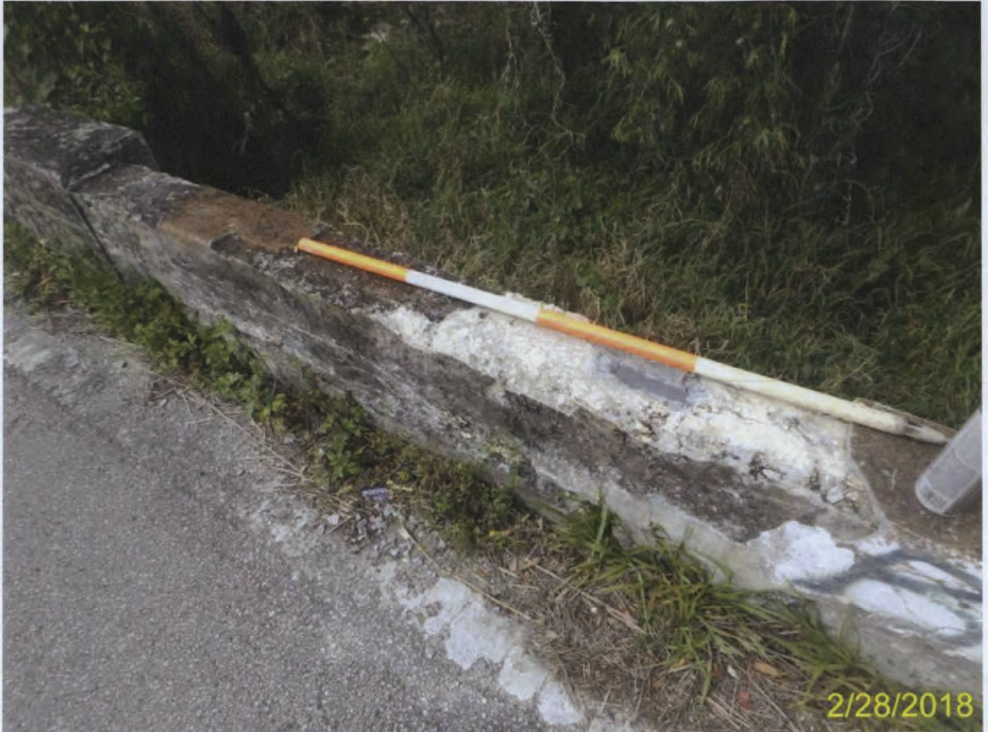
Photo 11 - Element 331 Re Conc Bridge Railing
