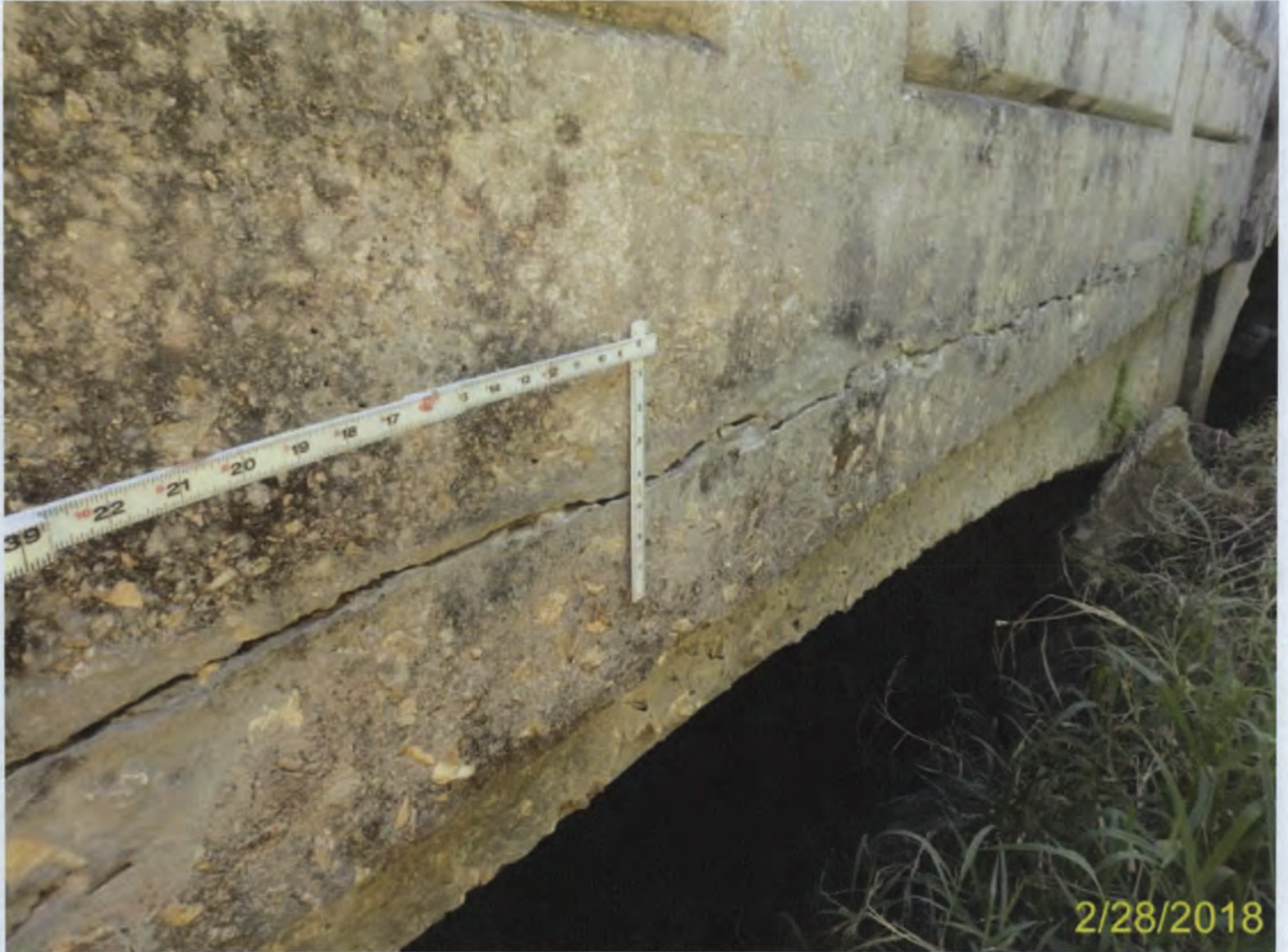
Photo 10 - Element 331 Re Conc Bridge Railing
