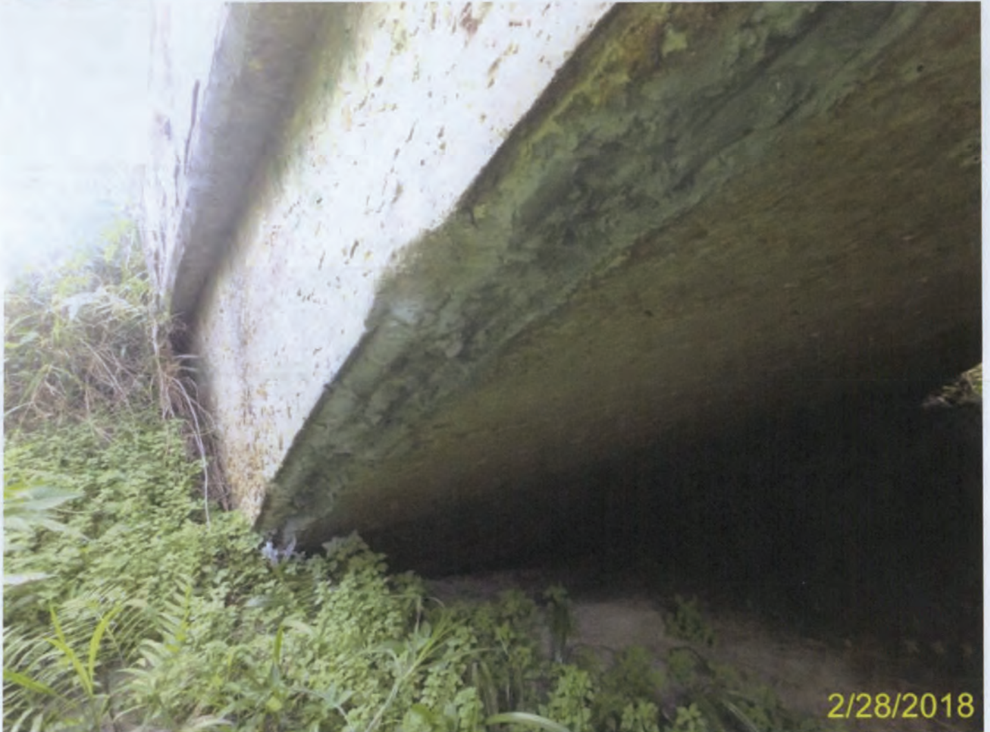
Photo 7 - Element 144 Re Conc Arch
