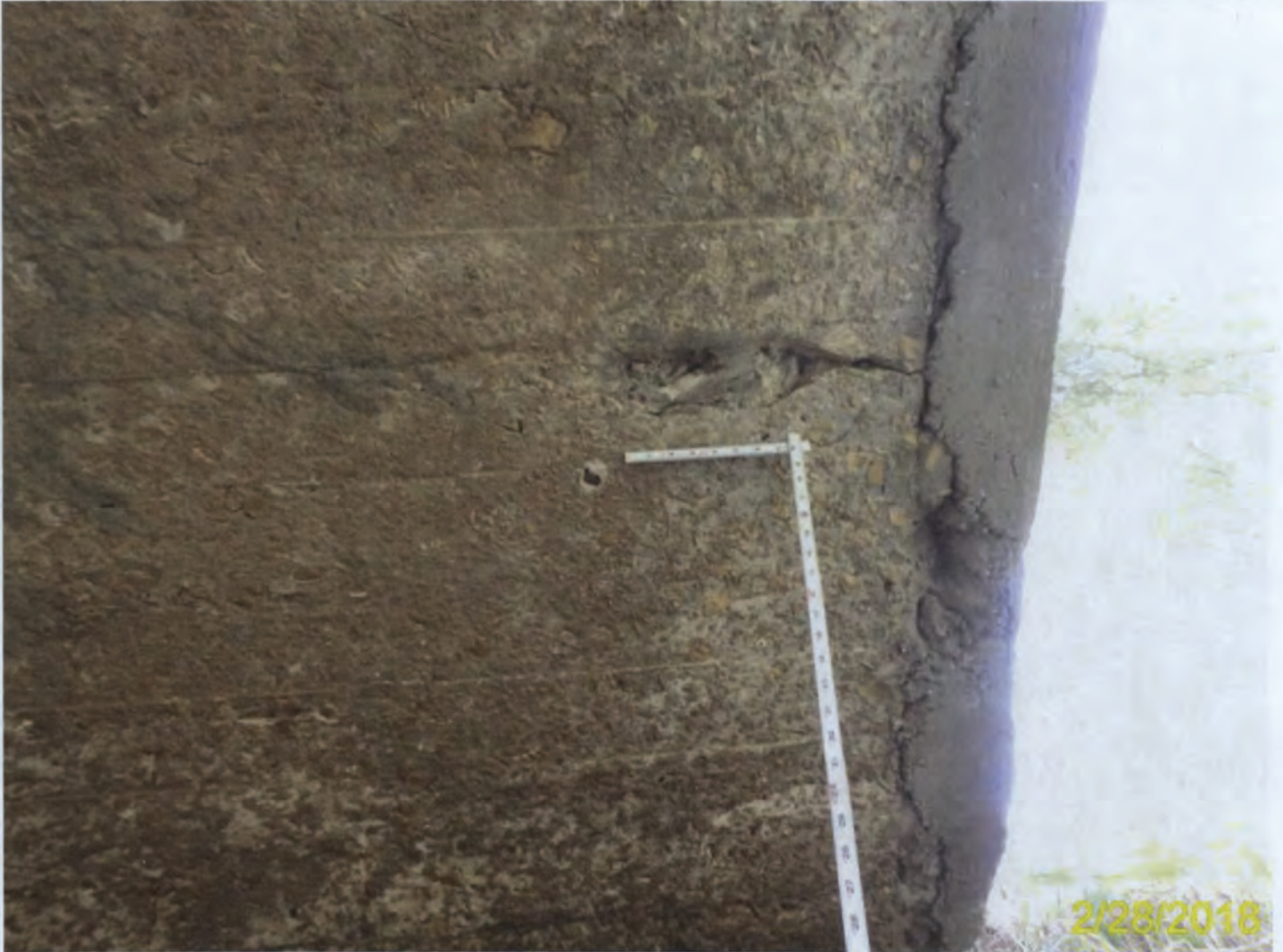
Photo 8 - Element 144 Re Conc Arch
