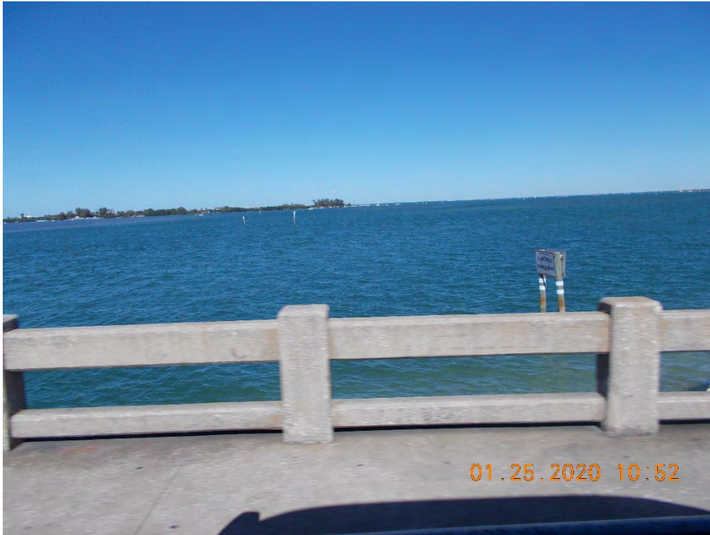
Photo 6B Bridge # 170022 – CSER Site #5.
