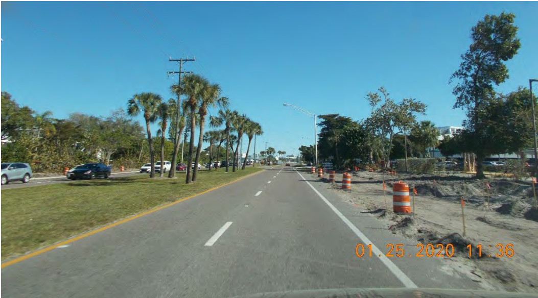
Photo 3C: Sidewalk Construction Area – CSER Site #2.
