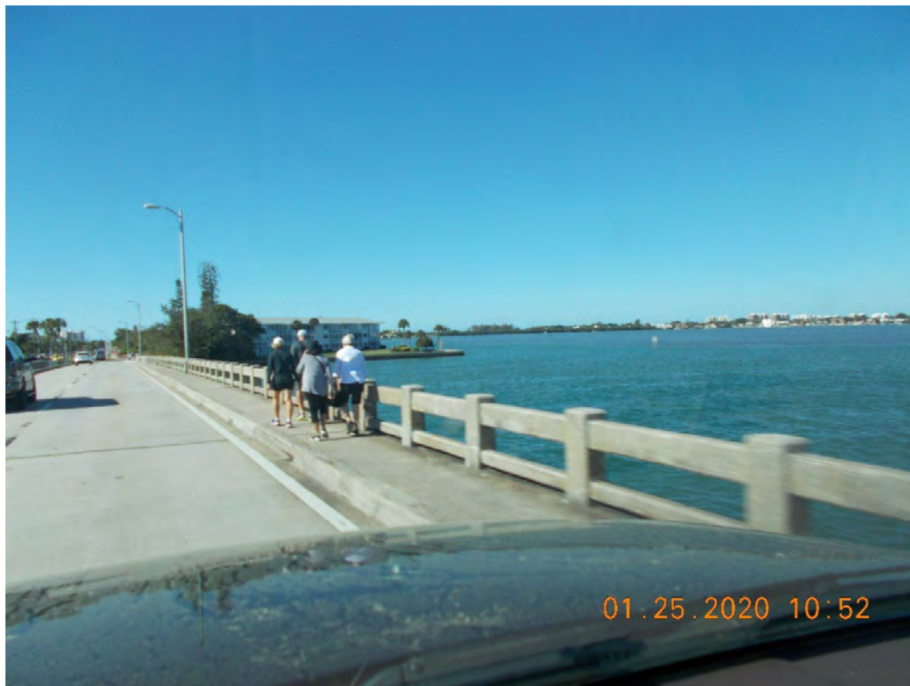
Photo 6A: Bridge # 170022 – CSER Site #5. View is Southbound.
