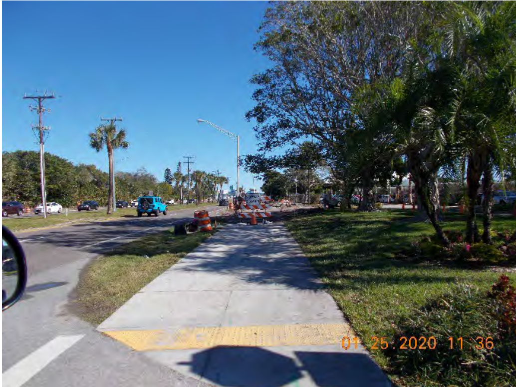
Photo 3B: Sidewalk Construction Area – CSER Site #2.
