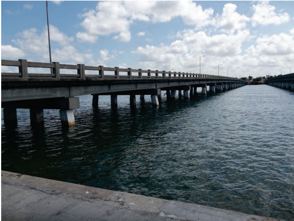
PHOTO 2 – 5/12/15 – VIEW OF SUPPORT PILES WITH PILE JACKETS
