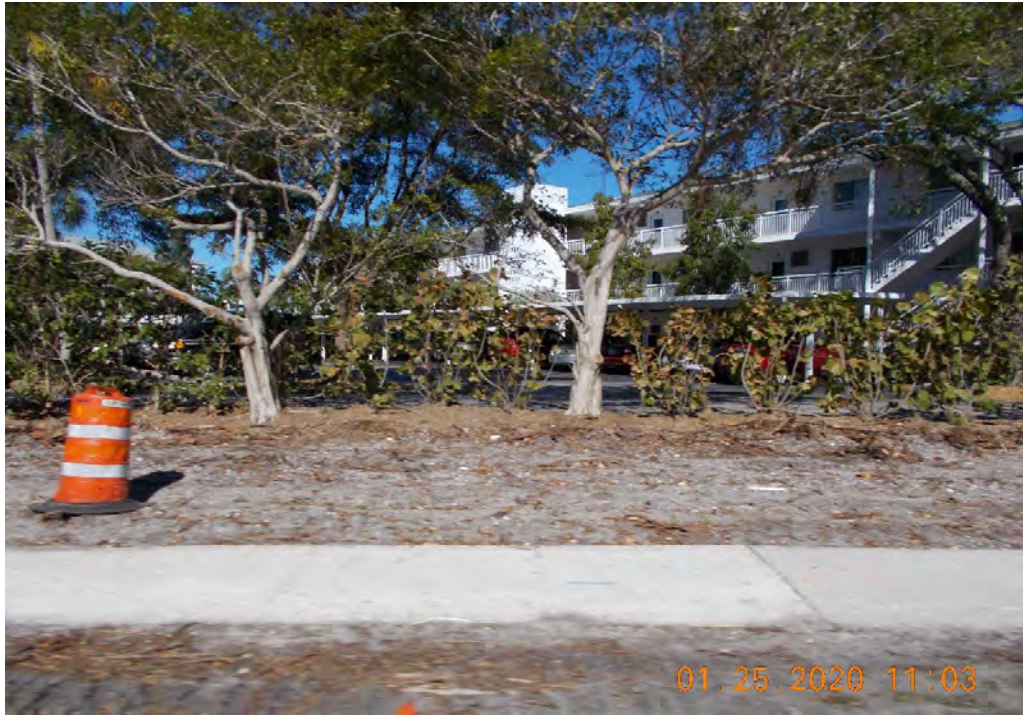
Photo 3A: Sidewalk Construction Area – CSER Site #2.
