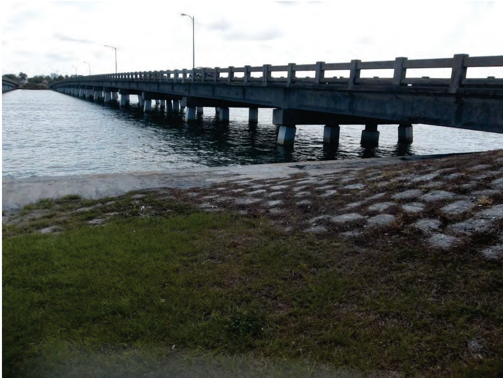
PHOTO 2 – 5/13/15 - VIEW OF SUPPORT PILES WITH PILE JACKETS
