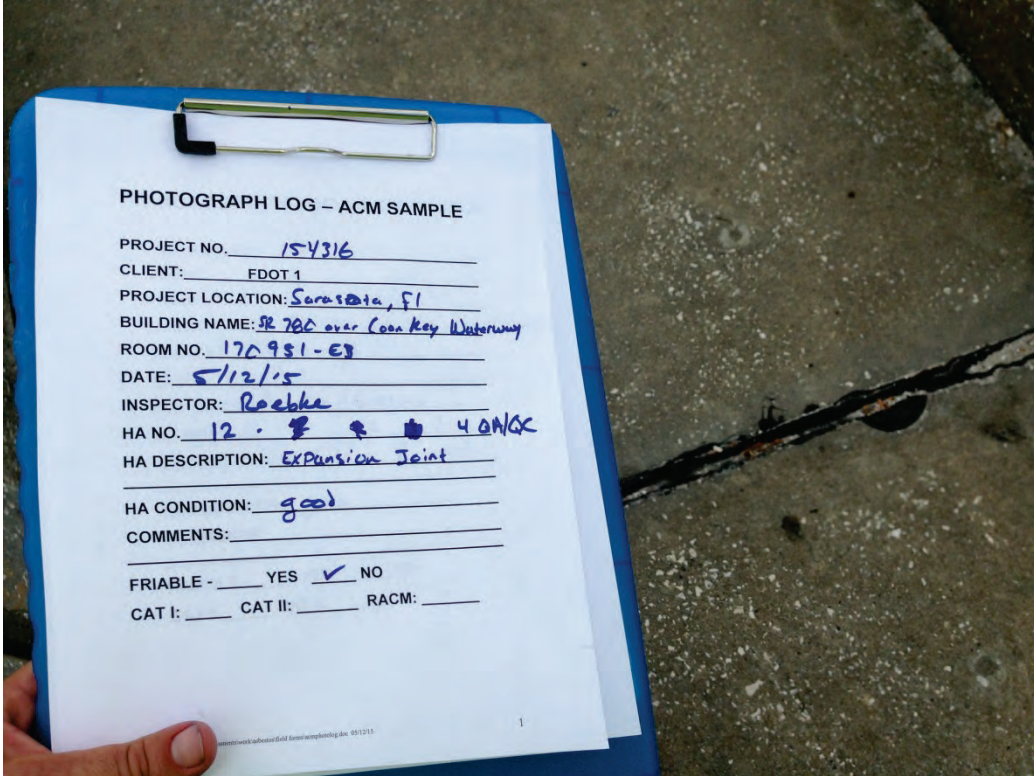
PHOTO 41 – 5/12/15 – SAMPLE 12.4 QA/QC – HA 12 RUBBER CAULKING EXPANSION JOINT
