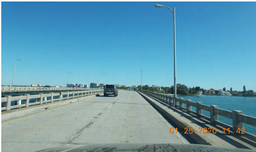
Photo 6C: Bridge # 170951 – CSER Site #5. View is northbound.
