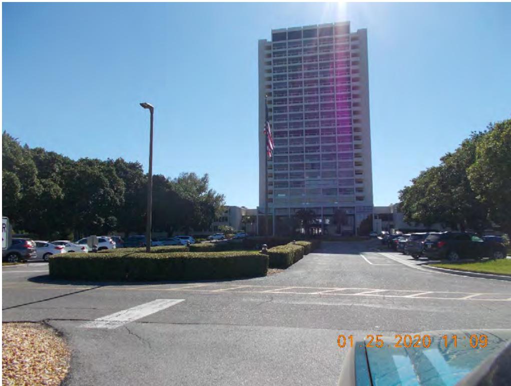
Photo 8A: Plymouth Harbor Retirement Community – CSER Site #7.
