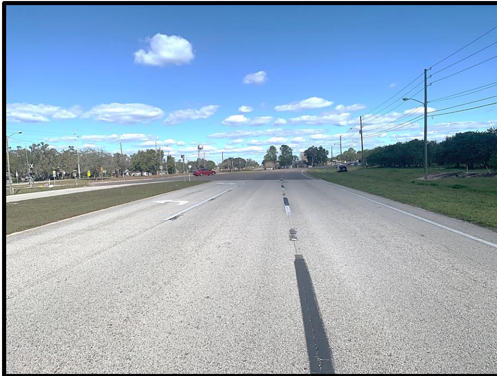
Looking North Towards Intersection
