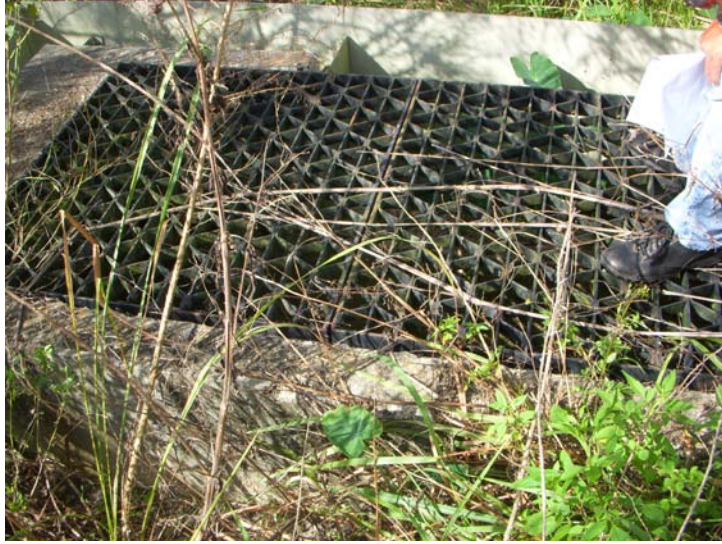
Upstream Control Structure
