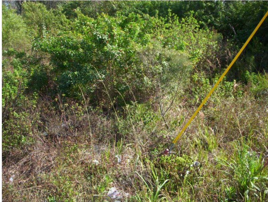
Upstream (Culvert not accessible due to vegetation)
